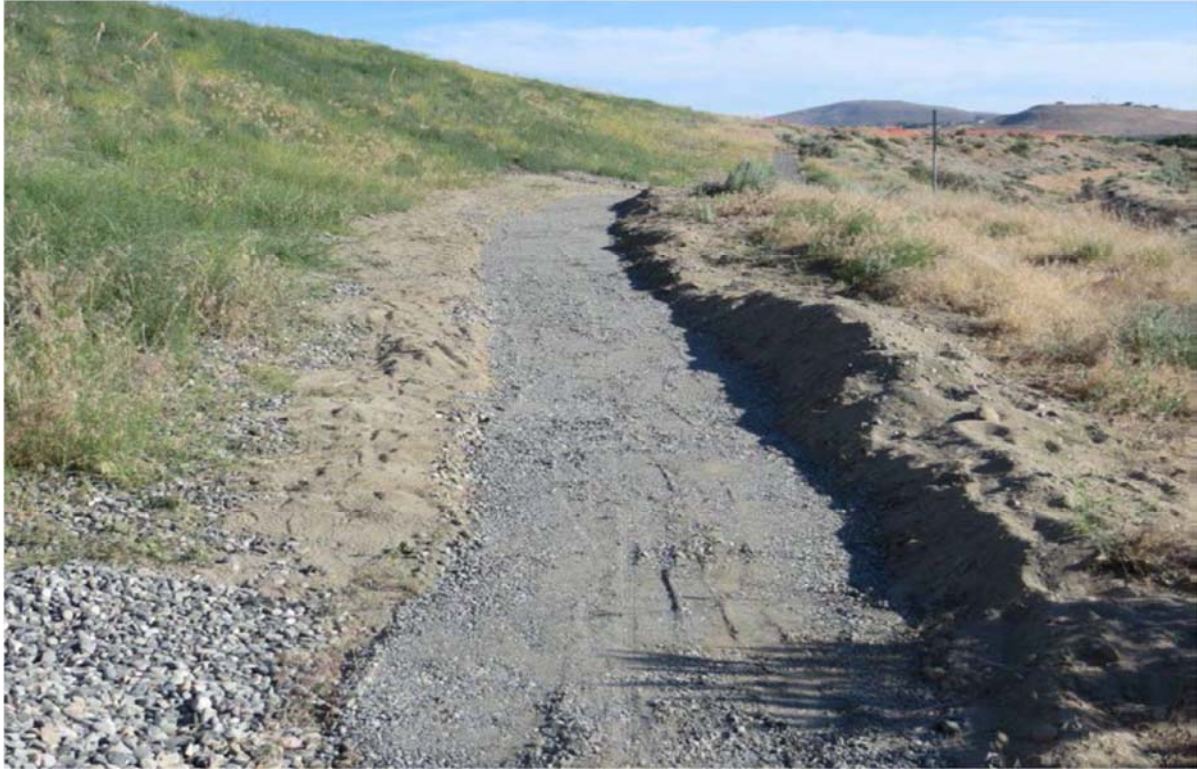
Figure 8. An Example of Finished Trail with 5/8 Inch Gravel Surface.
