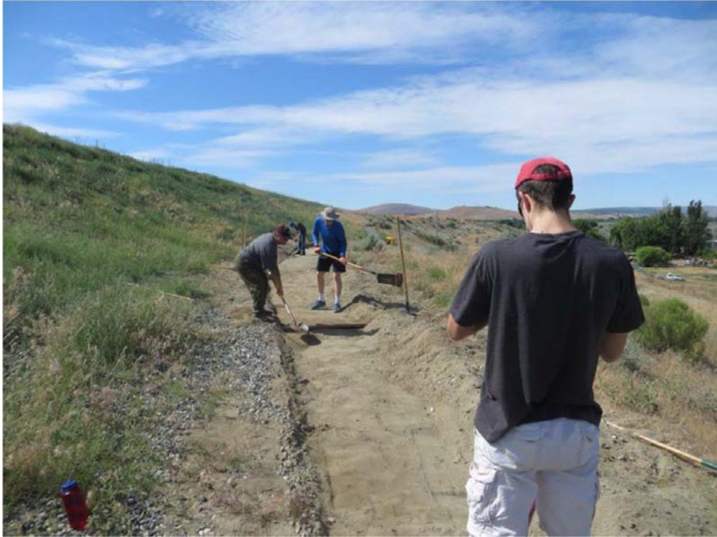
Figure 6. An Example of Initial Trail Preparation Consists of Excavating Approximately 6-Inches Below Surface.
