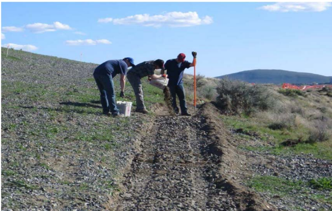
Figure 7. An Example of Spreading the Ballast Rock along the Trail Subsurface.
