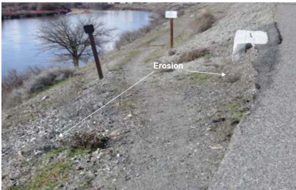
Figure 3. Unstable Slope at the Start of the Trail.
