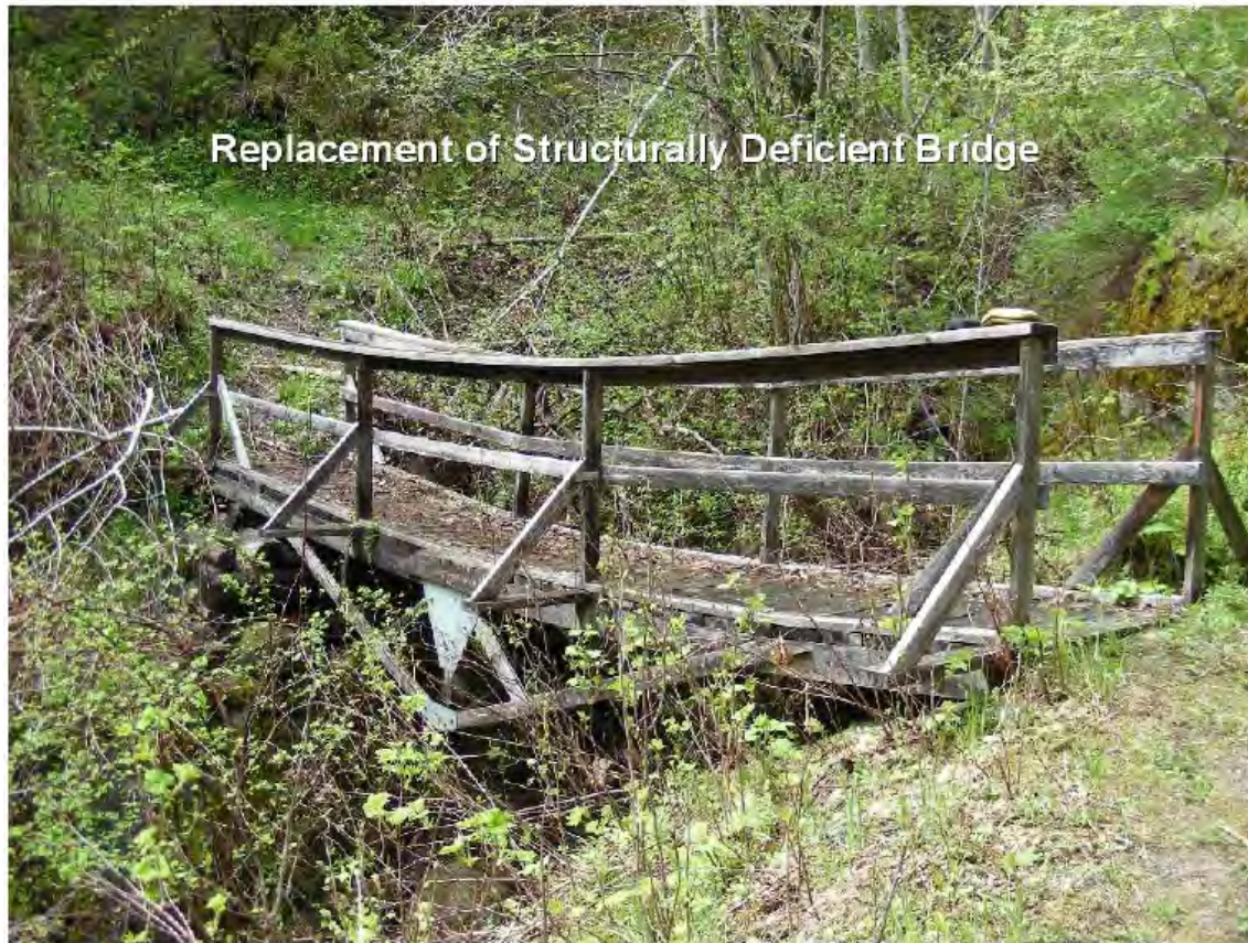
Figure 5 Typical bridge on recreation trails at Dworshak.
