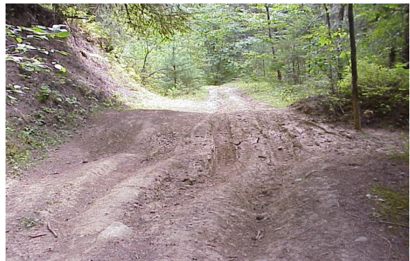
Photos 3-7 and 3-8. The effects of ATV use on undesigned, undeveloped trails on Dworshak
