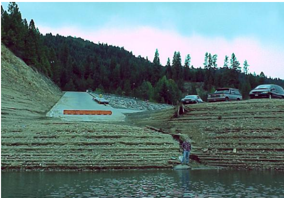
Photo 3-3. Boat Launch Ramp and Parking.
