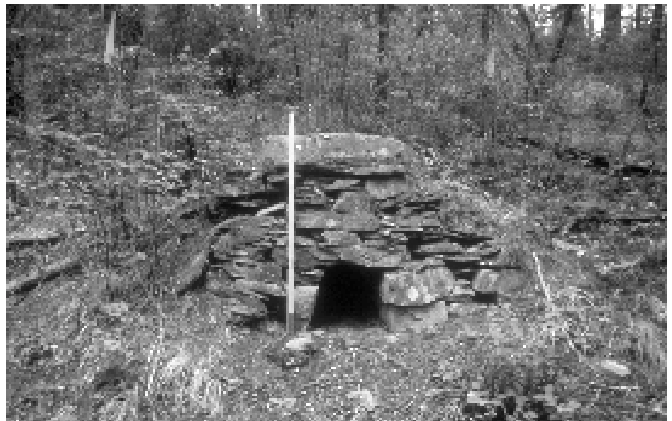
This stone structure (c. 1905) is one of three bread ovens associated with the Spokane and International Railroad Construction Camp near Eastport (Boundary County). All that remains of the temporary railroad camp are building depressions, log wall remnants, dumping areas, and these ovens, believed to be erected by Italian construction laborers. (c. 1990; ISHS 1997.21.7.)
