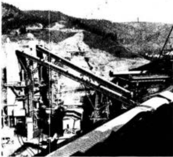
BATCH PLANT AND OVERHEAD CABLEWAY TAKEN FROM AGGREGATE AREA.
