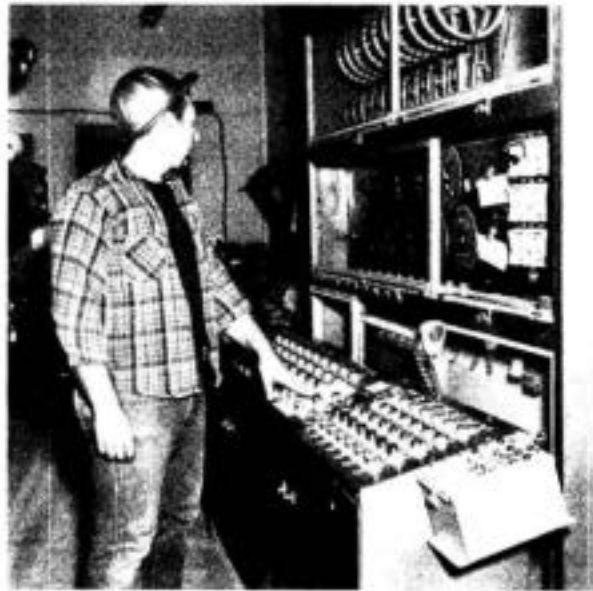
BATCH PLANT CONTROLS.
