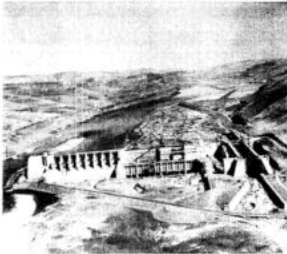
1st-STEP CONSTRUCTION - SEP 1968
