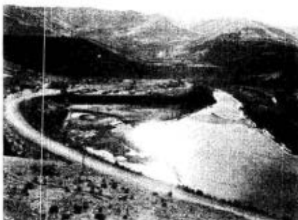
DIVERSION CHANNEL CLOSED; DAM CONSTRUCTION UNDERWAY
