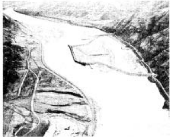
COFFERDAM & DIVERSION COMPLETE DECEMBER 1966
