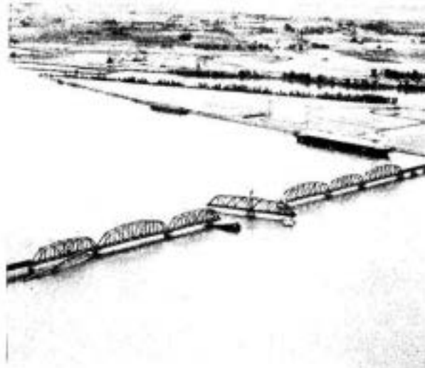
UPRR BRIDGE BELOW SNAKE RIVER (TO BE REPLACED)
