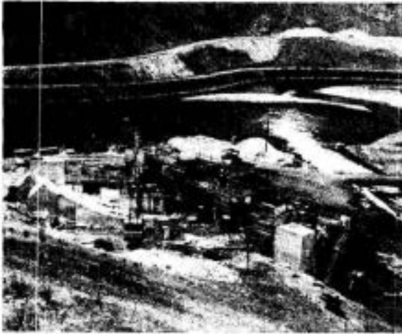
OUTLET WORKS WITH FLIP BUCKETS ON LEFT
