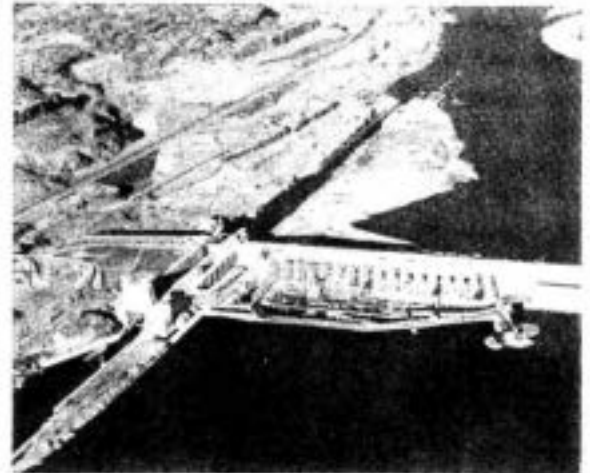
RAISING LOW SPILLWAY BAYS - 1967
