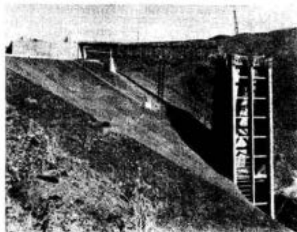
INTAKE TOWER FOR OUTLET WORKS; SPILLWAY ON LEFT; DAM ON RIGHT
