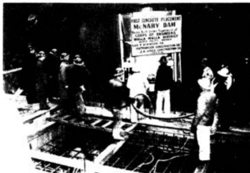
FIRST CONCRETE POUR - IN NAVIGATION LOCK - 15 DECEMBER 1948
