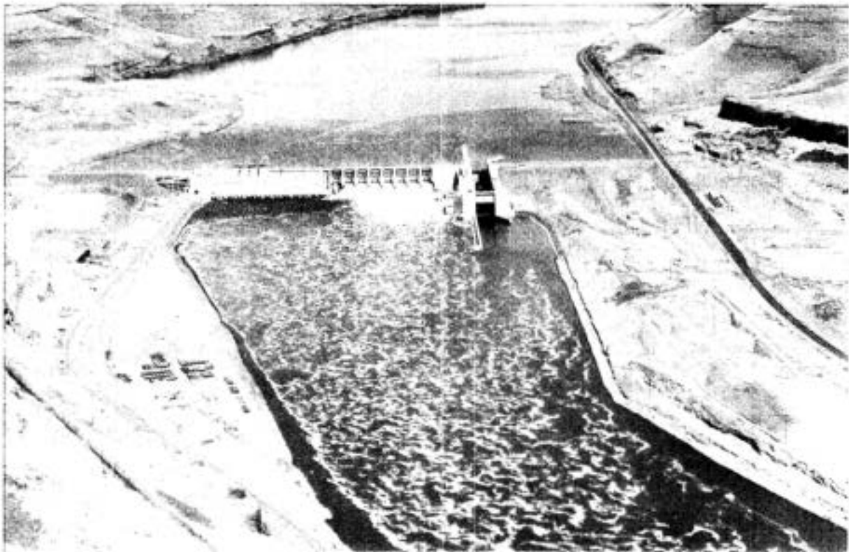
LOWER MONUMENTAL DAM - RIVER MILE 41.6
