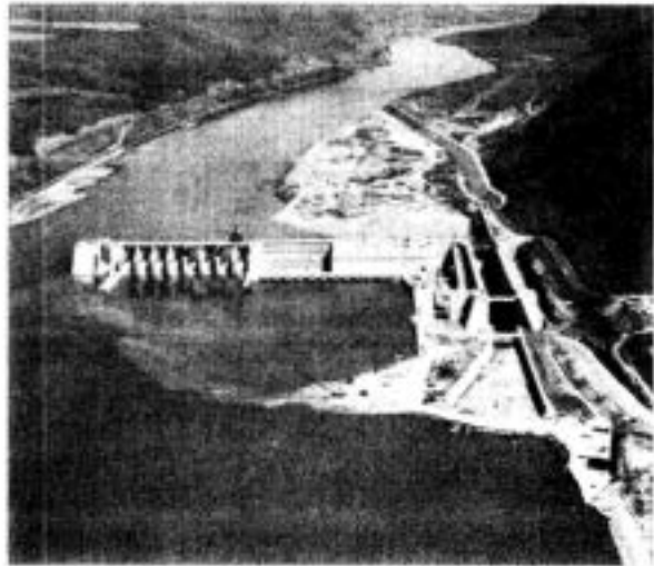
COFFERDAM OUT - MAY 1969
