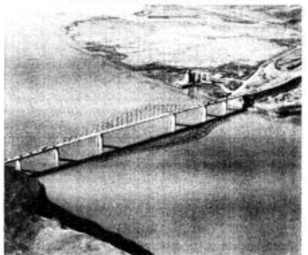
CENTRAL FERRY STATE PARK AREA NORTH SHORE BELOW BRIDGE
