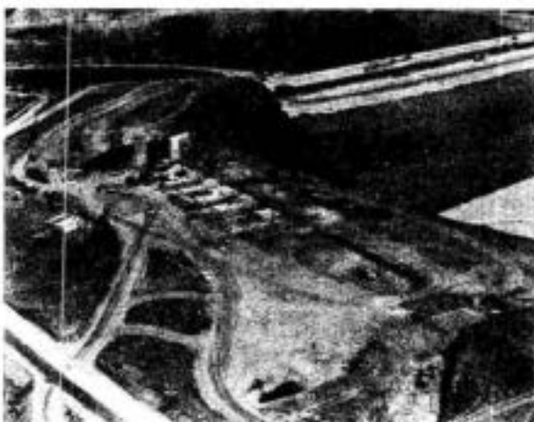
SPILLWAY CREST UNDER CONSTRUCTION
