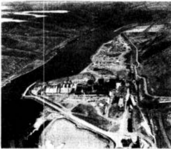
1st-STEP COFFERDAM - OCT 1968
