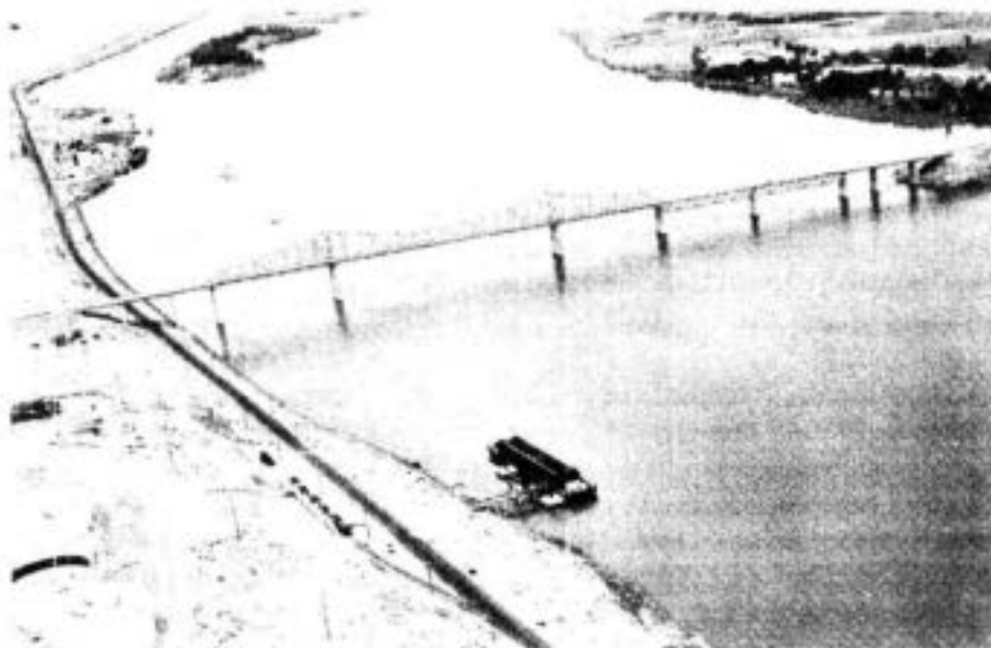
NEW SNAKE RIVER HIGHWAY BRIDGE
