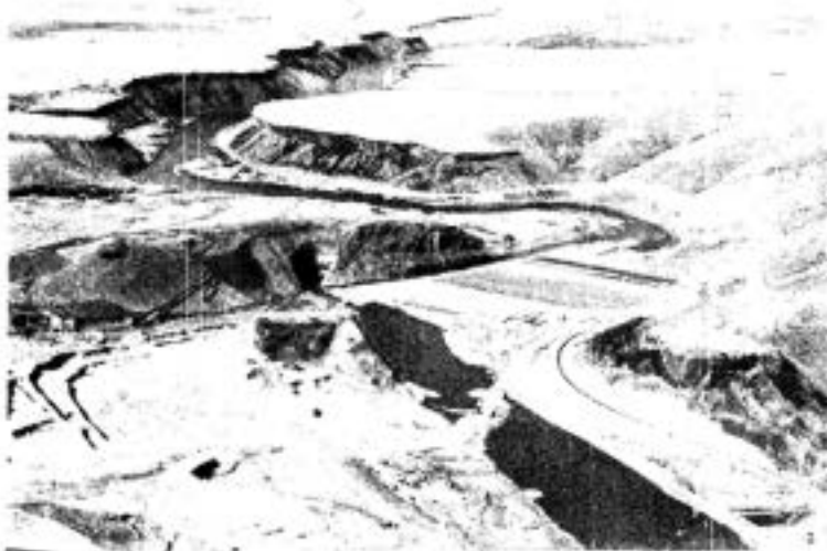
LUCKY PEAK DAM CONSTRUCTION OCT 1951 LOOKING DOWNSTREAM--BOISE IN UPPER RIGHT
