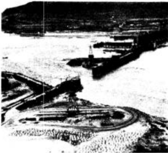
OREGON SHORE COFFERDAM READY TO CLOSE GAP IN CELLS NOTE TETRAHEDRONS IN FOREGROUND
