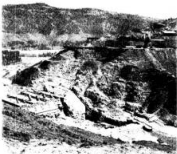
RELATION OF BATCH PLANT TO TRAMWAY AND CONSTRUCTION SITE.
