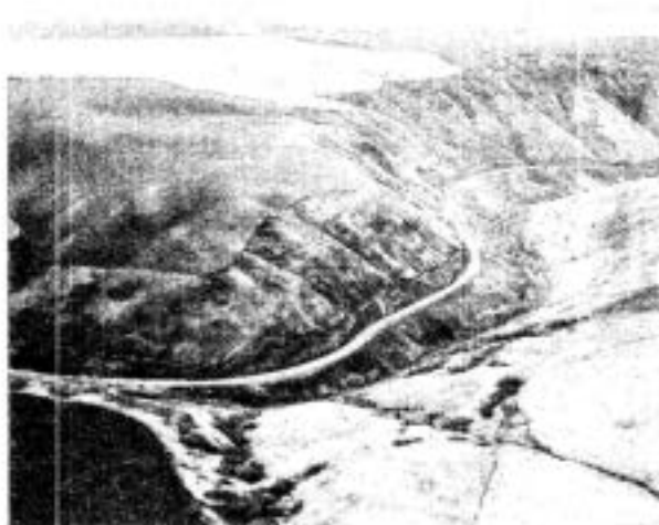
ACCESS ROAD - POMEROY TO DAM DECEMBER 1966
