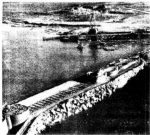
CLOSURE SECURE - READY FOR CRIB SUPERSTRUCTURE
