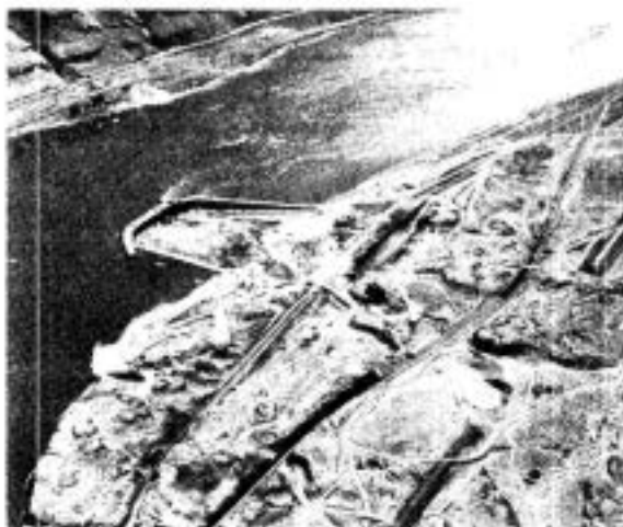
1st STEP CONSTRUCTION - 1959
