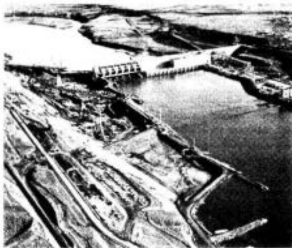
SECOND STEP - NORTH SHORE COFFERDAM WORK - 1960
