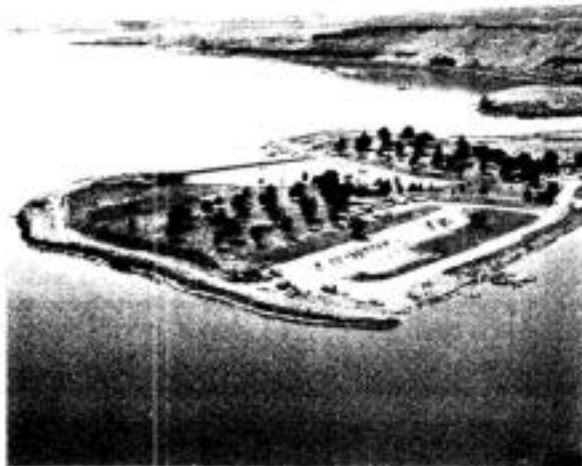
LEVEY PARK - BOATING, SWIMMING, AND PICNICKING FACILITIES
