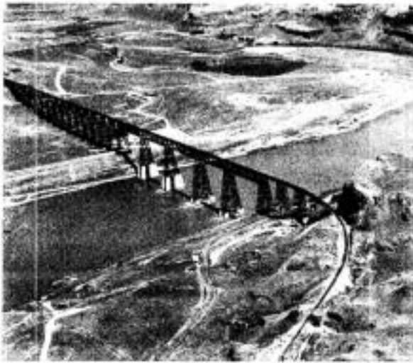
UPRR - JOSO BRIDGE
