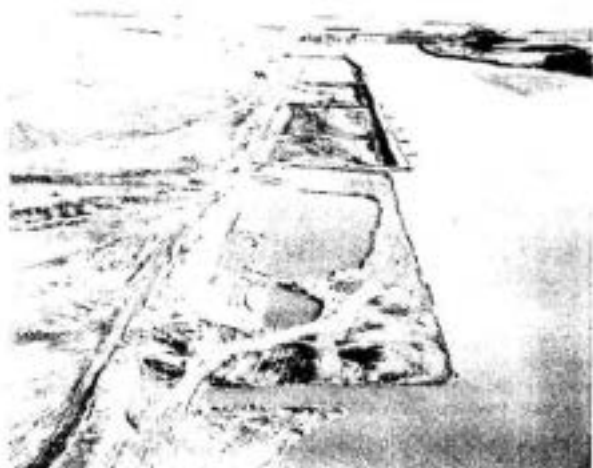
DOWNSTREAM NAVIGATION CHANNEL EXCAVATION
