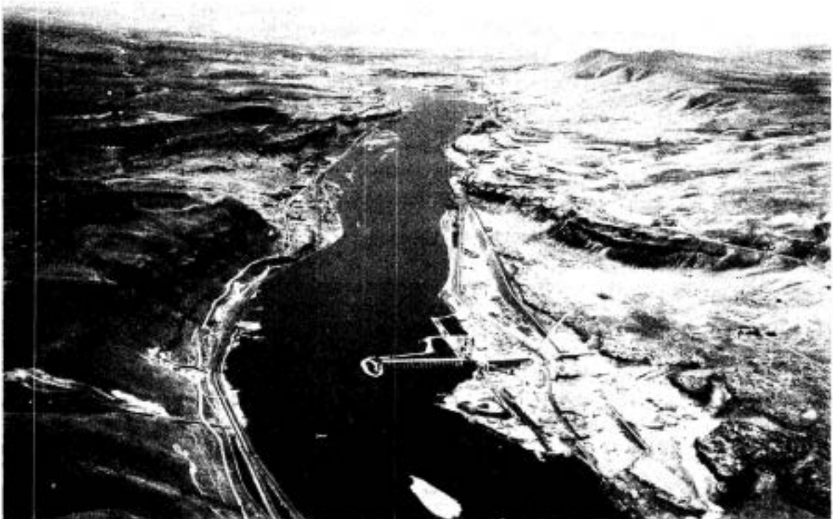
JOHN DAY DAM SITE AREA LOOKING WEST WITH MT. HOOD IN BACKGROUND
