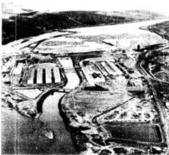
PFI COMPLEX - PLANT, LOG POND, AND WWP DAM ON CLEARWATER RIVER
