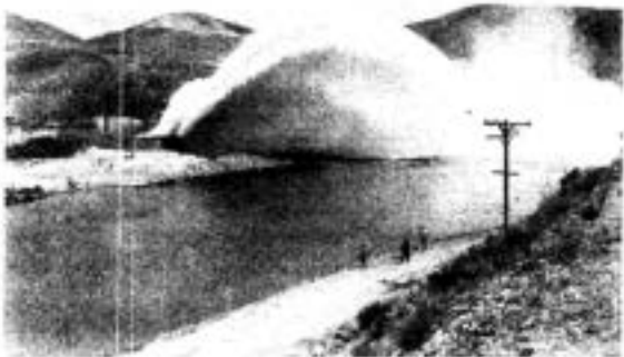
OUTLET WORKS IN OPERATION
