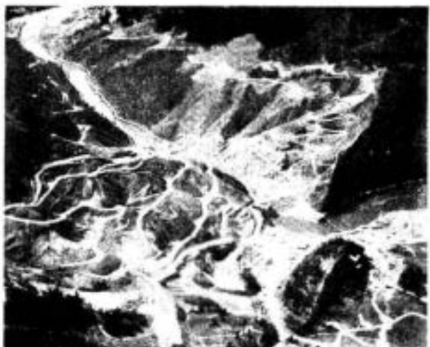
DWORSHAK DAM - APRIL 1967
