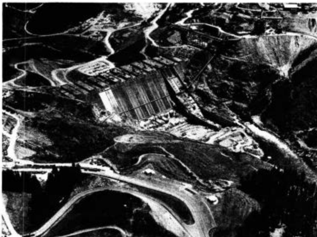
CLOSE TO FOUR MILLION CUBIC YARDS CONCRETE IN PLACE. BATCH PLANT UPPER RIGHT CORNER. SPILLWAY CENTER OF PICTURE WITH POWERHOUSE STARTING AT LEFT TOE OF DAM. DIVERSION TUNNEL AND FISH TRAP RIGHT CENTER. BYPASS ROAD AND VISITOR OVERLOOK HOUSES IN LOWER CENTER.
