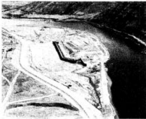
START OF COFFERDAM & RIVER DIVERSION LOOKING UPSTREAM - JUNE 1966
