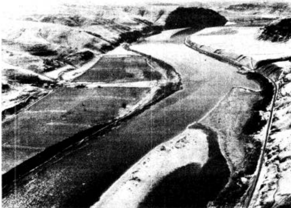
SNAKE RIVER - LOOKING DOWNSTREAM AT LITTLE GOOSE DAMSITE. DAM TO SPAN RIVER AT BUILDINGS ON LEFT. RIPARIA RAILROAD BRIDGE IN BACKGROUND.
