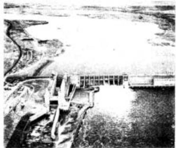
PARTIAL POOL - READY TO REMOVE SECOND STEP COFFERDAM - JAN 1962
