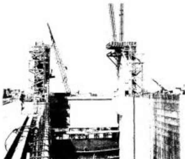
LOWER NAVIGATION LOCK GATE CONSTRUCTION WITH COUNTERWEIGHT TOWERS, NOTE ALSO THE NORTH SHORE FISHWAY ENTRANCE AND LADDER
