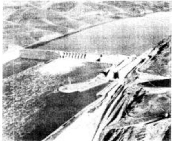
NORTH SHORE EMBANKMENT AND POOL UP - 19 FEB 70
