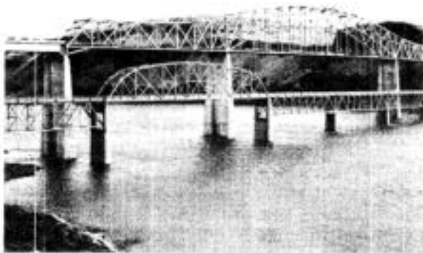
OLD AND NEW CENTRAL FERRY BRIDGE
