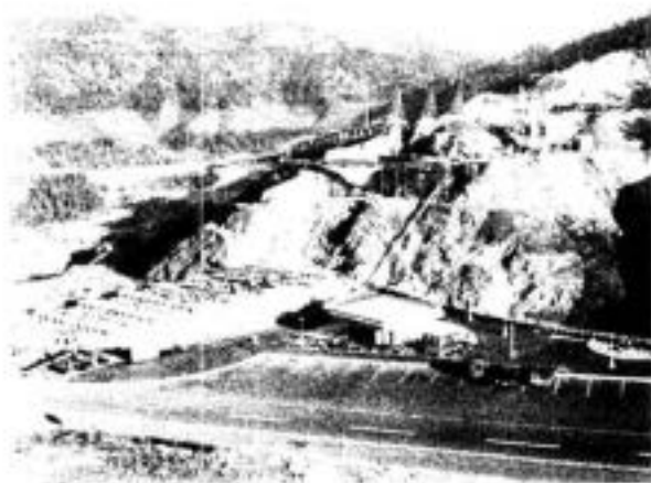
VISITORS' OVERLOOK AREA AND VIEW OF CONSTRUCTION AREA
