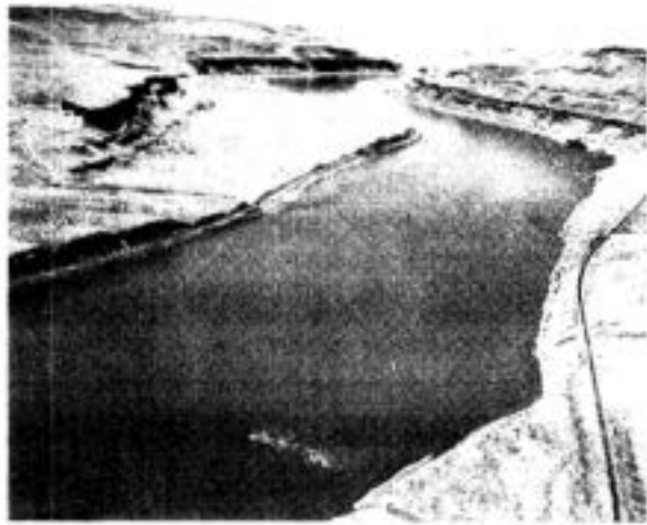
THE DAMSITE (LOOKING WEST - DOWNSTREAM)
