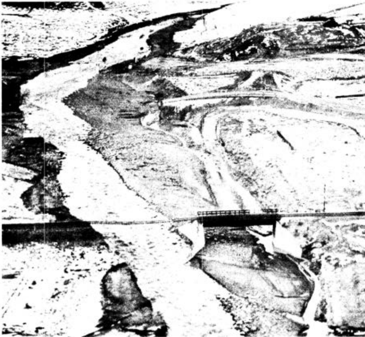
HIGHWAY AND RAILROAD DESTRUCTION AT ALDER CREEK CANYON, WASHINGTON
