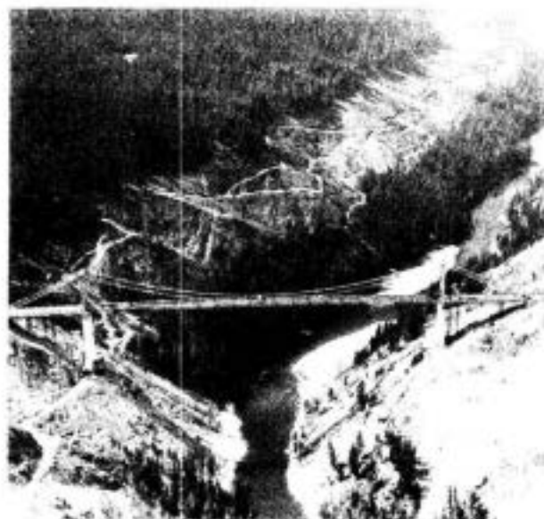
DENT BRIDGE FOR ACCESS FROM WEST SIDE TO OROFINO LOOKING DOWNSTREAM
