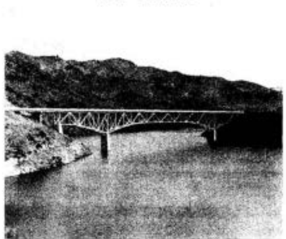
MORES CREEK BRIDGE AND RESERVOIR
