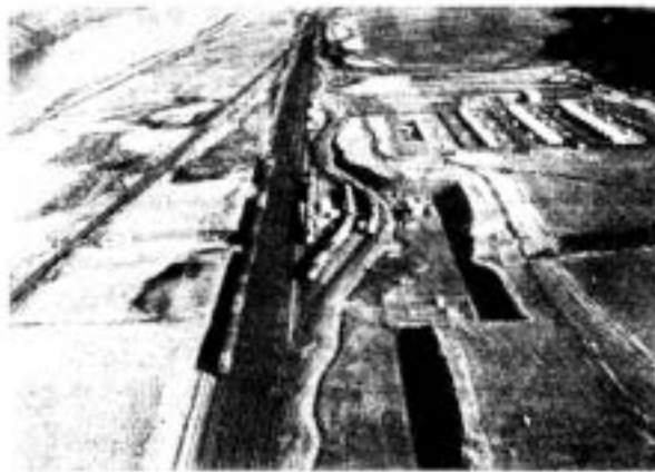
UPRR-RELOCATED AYER TOWNSITE & LINE
