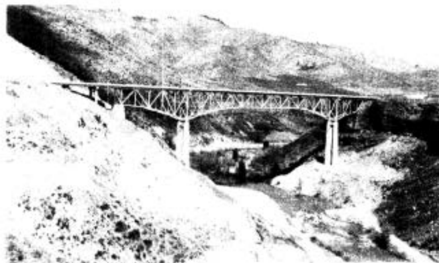
MORES CREEK BRIDGE 1954 LOOKING UPSTREAM BEFORE POOL RAISING
