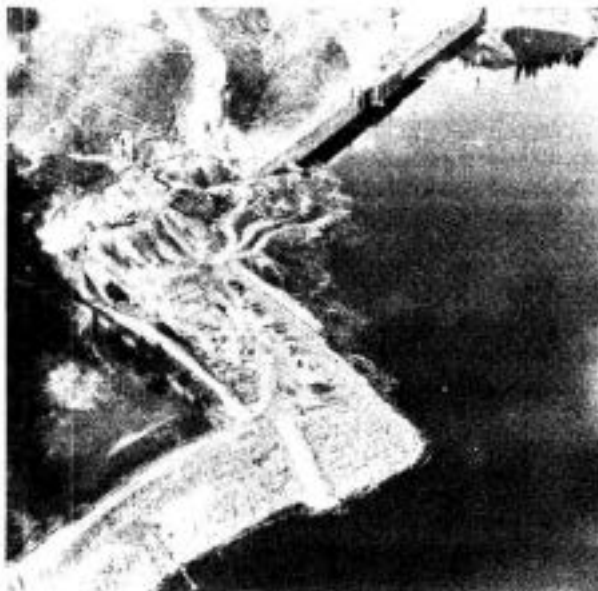
LOG HANDLING AREA AT LEFT ABUTMENT POOL PARTIALLY RAISED WITH CONSTRUCTION STILL IN PROGRESS
