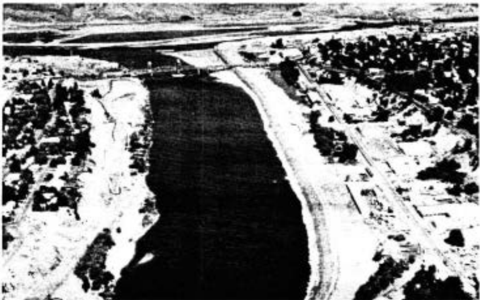
SNAKE RIVER - LEWISTON WATERFRONT LEVEE Interstate Bridge and Mouth of Clearwater River in Background Clarkston Washington - Left Bank
