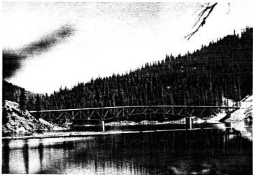
GRANDDAD BRIDGE (River Mile - 40)
