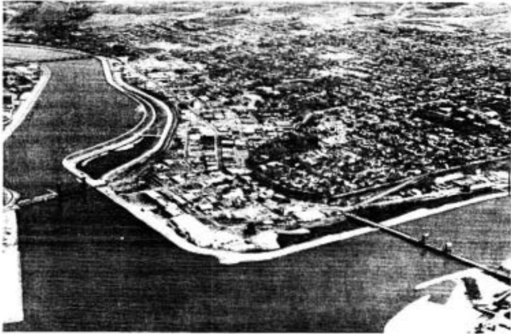
LOWER GRANITE RESERVOIR - LEWISTON WATERFRONT Interstate Bridge Right Foreground - Memorial Bridge Left Background
