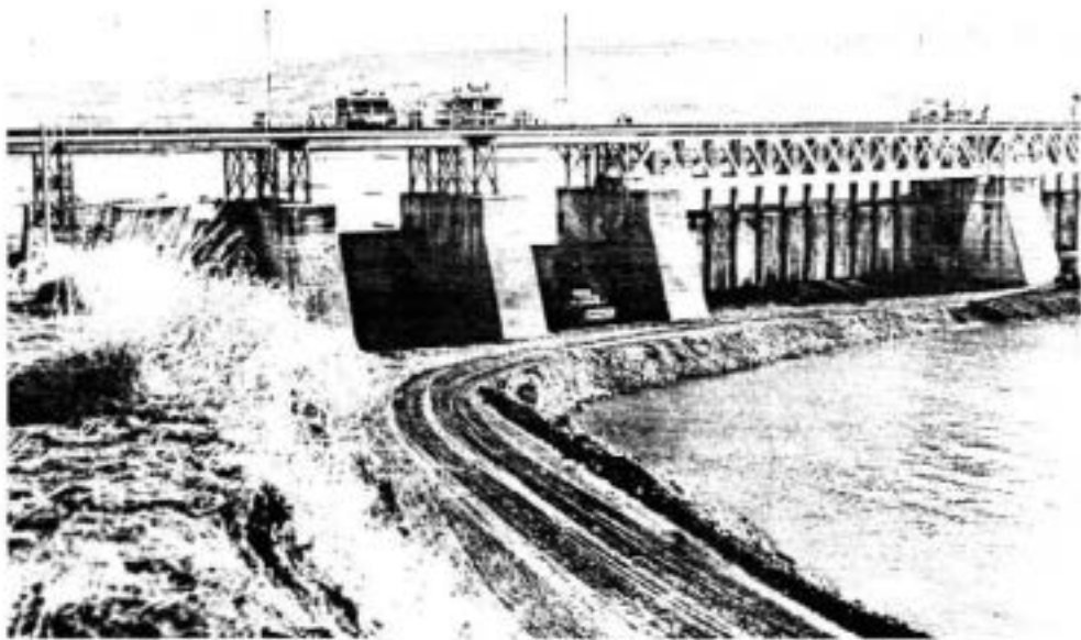
REMOVAL WASHINGTON WATER POWER DAM
