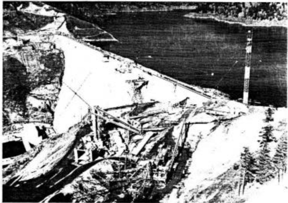
CONSTRUCTION PROGRESS February 1973 Powerhouse at Toe of Dam
