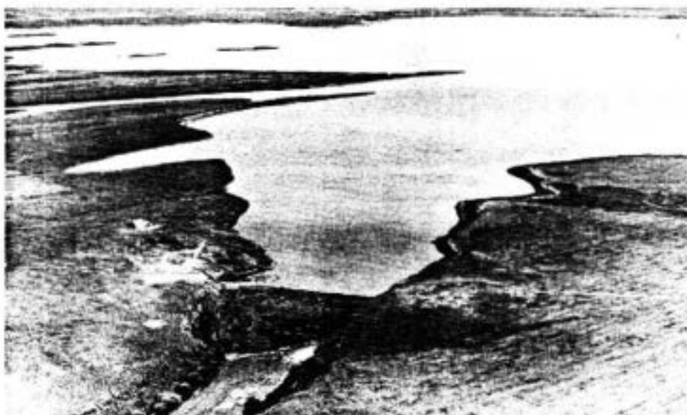
Existing Blackfoot Dam - Looking Up- stream. Dam and Spillway Outlet Works on Right
