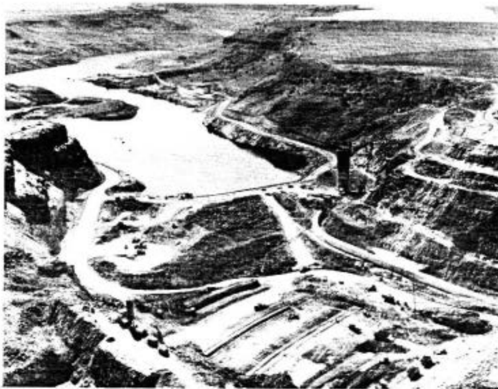
RIRIE DAM CONSTRUCTION - SEPTEMBER 1974 Spillway Channel, Left Foreground; Dam, Downstream Face; and Outlet Conduits
