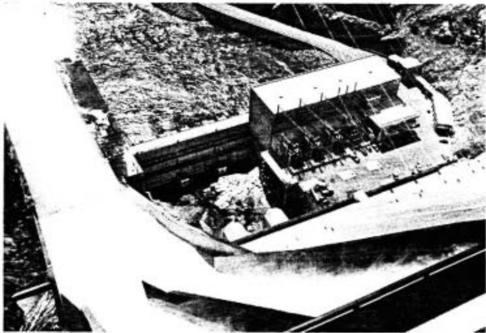
POWERHOUSE JULY 1974 Future Unit Space Center of Picture Spillway at Left
