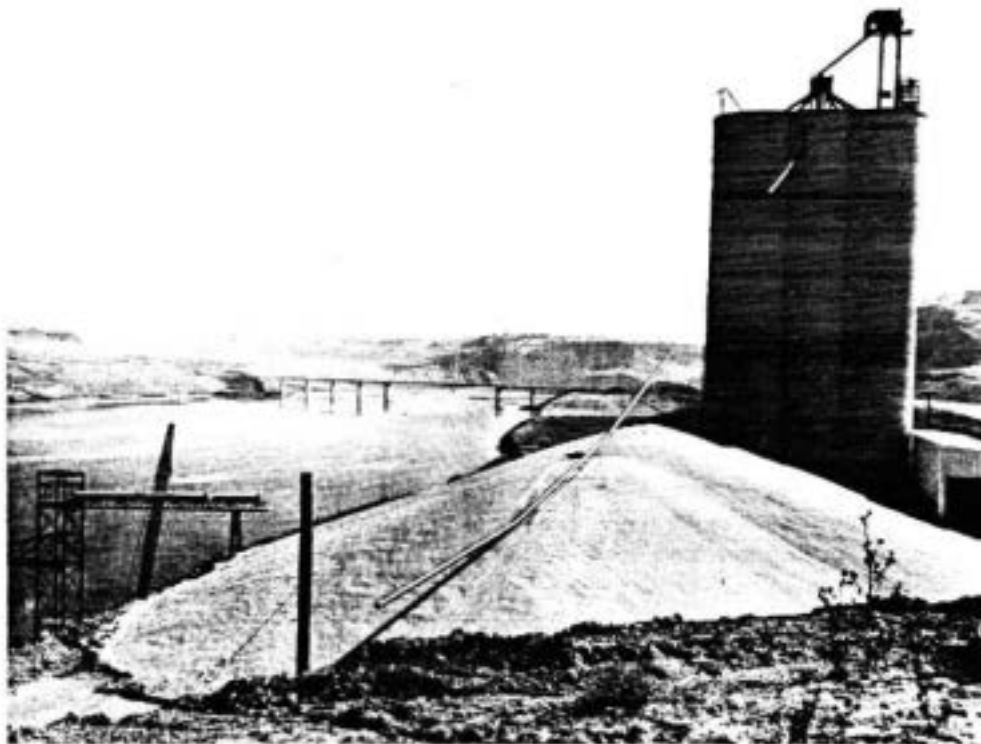
PORT OF COLUMBIA COUNTY Wheat Storage Awaiting Shipment
