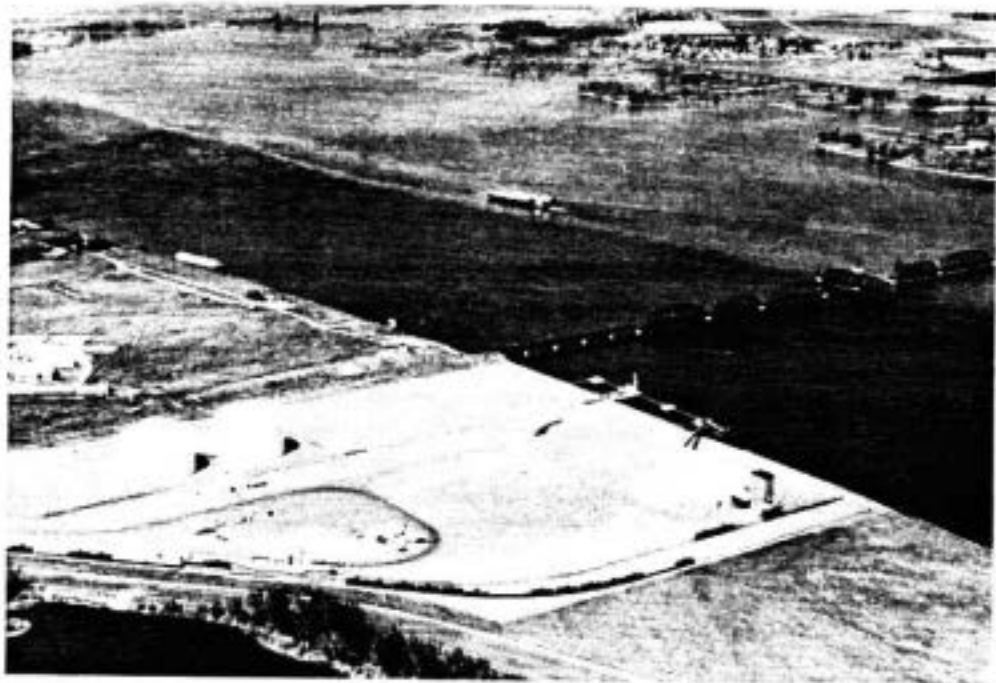
UPRR BRIDGE NPRR Bridge at Mouth of Snake River in Background
