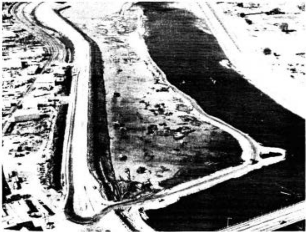
CLEARWATER RIVER - MEMORIAL (16TH STREET) Bridge Downstream - Levee and By-Pass Road Along Lewiston Waterfront Holbrook Island Excavation Center of Picture North Bank Levee in Place
