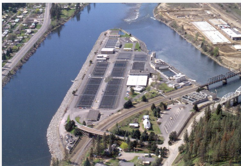
Photo 1. Aerial View of DNFH
