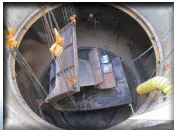
Walla Walla District's maintenance crews from the McNary project rigged and picked the first half of the diffuser ring from fish pump #2 for temporary storage on May 18. After a pre-critical lift meeting prior to, the operation went smoothly. The rotor was removed to access lower components which were in need of repair. (Photos by Terry Zerby)
