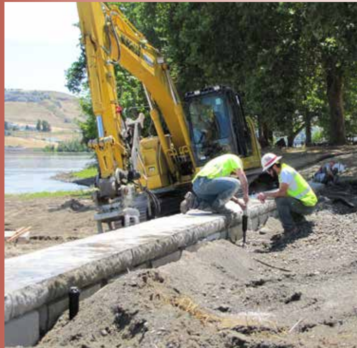
Above and Right: U.S. Army Corps of Engineers Maintenance Worker Jeremiah Harris puts the finishing touches on a new life-ring station at the Chestnut Recreation Area in Clarkston, Washington. The area was temporarily closed May 31 to enable maintenance staff to replace a 240-foot-long dilapidated rock-and-mortar wall (right), which was falling apart and beginning to pose a safety risk to visitors. Corps staff originally estimated the work would continue until mid-August, but thanks to cooperative weather and ideal work site conditions, the project was completed early. (U.S. Army Corps of Engineers photos by John Gordon)
