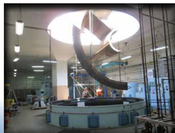
Walla Walla District's maintenance crews from the McNary project rigged and picked the first half of the diffuser ring from fish pump #2 for temporary storage on May 18. After a pre-critical lift meeting prior to, the operation went smoothly. The rotor was removed to access lower components which were in need of repair. (Photos by Terry Zerby)
