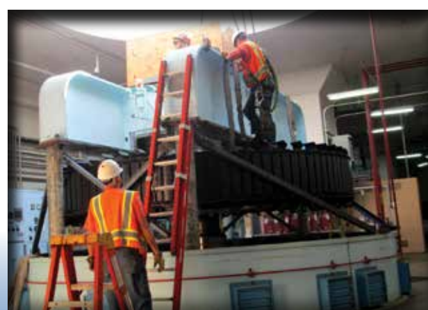
Walla Walla District's maintenance crews from the McNary project rigged and picked the first half of the diffuser ring from fish pump #2 for temporary storage on May 18. After a pre-critical lift meeting prior to, the operation went smoothly. The rotor was removed to access lower components which were in need of repair. (Photos by Terry Zerby)
