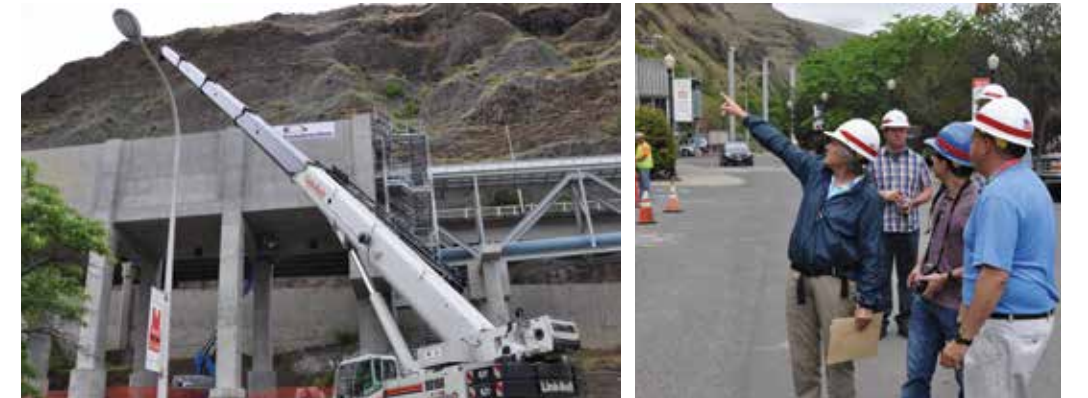
Left Page: Contractors and Corps Employees continue to work to improve the Juvenile Bypass System (JBS) at Lower Granite Dam. The illustration above shows the changes being made to the JBS. Left: Construction continues at the JBS to 'daylight' incoming juvenile fish. Above Right: Fish Biologist Ann Setter answers questions at the JBS 'media day.' (Photos by Bruce Henrikson)
