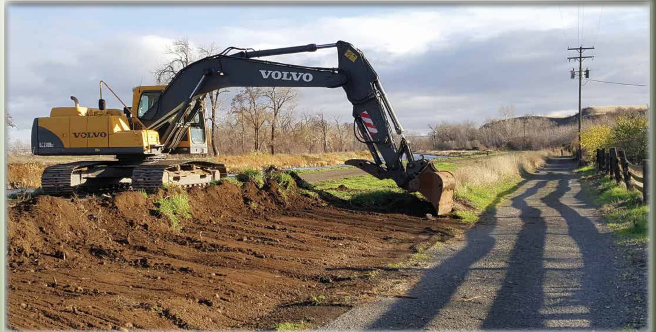
The contractor performs an initial surface grubbing of the landside slope of the south levee (left bank) to remove the existing vegetation layer. The contractor started at the access gate and worked upstream, completing approximately 3,000 linear feet before the snow fell, postponing work.
