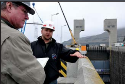
Project Manager Steve Thompson updates Walla Walla's Union-Bulletin Reporter Andy Porter on the navigation wall repair project during January's Lower Monumental public tour.
