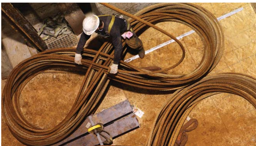
Contract workers replace Lucky Peak's intake tower wire rope in November 2010. (Inset) The District was also able to troubleshoot for future repairs of leaking valves while inspecting the dewatered intake tower.
