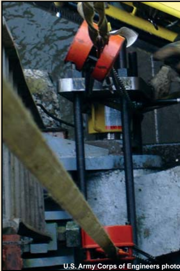
U.S. Army Corps of Engineers photo
