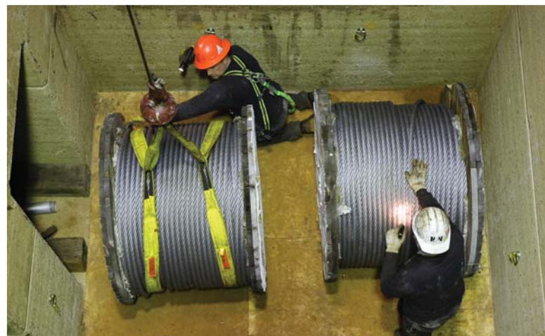
Contract workers replace Lucky Peak's intake tower wire rope in November 2010. (Inset) The District was also able to troubleshoot for future repairs of leaking valves while inspecting the dewatered intake tower.
