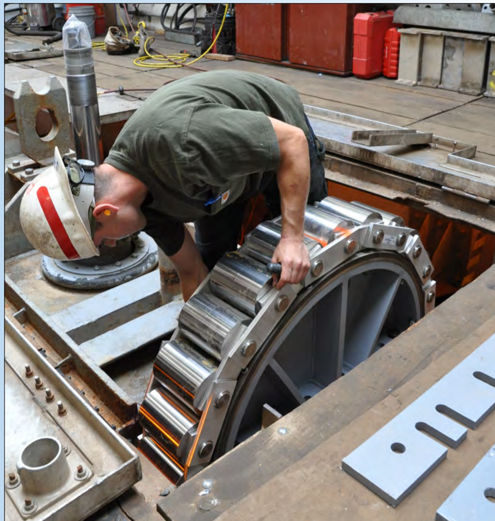
Above: Colbey Soule, a powerplant mechanic at McNary Lock and Dam, works on installing new roller chain onto a turbine headgate. More than 120 Walla Walla District employees work at the McNary Project. They serve as electricians, lock operators, painters, welders, riggers, utility workers, mechanics, biologists, environmental resource specialists, park rangers, heavy equipment operators, administrative staff, engineers and maintenance workers. Together, they support the safe and continuous operation of the project.
