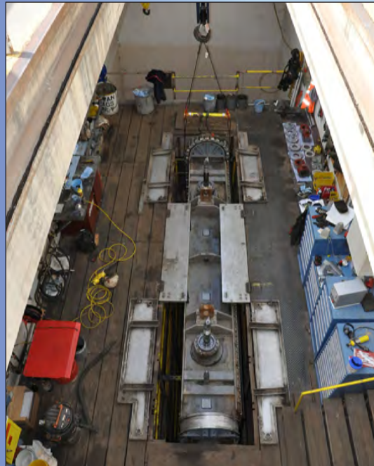
McNary Lock and Dam maintenance staff work inside one of the turbine headgate repair pits repairing the gates and associated parts to optimize performance and service life.
