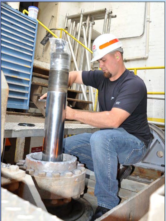
Rich Maldonado, McNary Lock and Dam powerplant mechanic worker-in-charge, works on reassembling rehabilitated parts of a turbine headgate.
