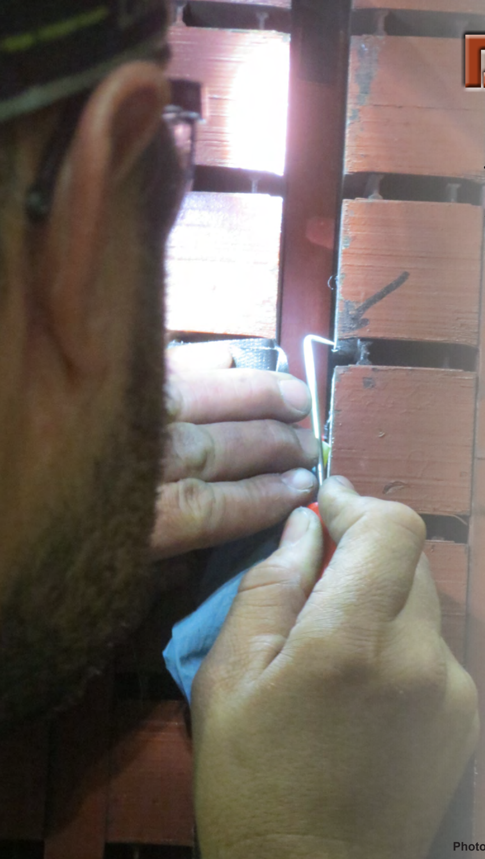
Left: Jesse Pearson cleans core lamination damage on Unit #3's stator winding. Right page clockwise: Dworshak Dam; Dworshak Dam Powerhouse; Workers perform a test braze on spare coils; Jesse Pearson (top) and Aaron Blackwell (bottom) unbrazed connections to the damaged stator winding; Chris Brown (left) and Jesse Pearson (right) pull the damaged coil.
