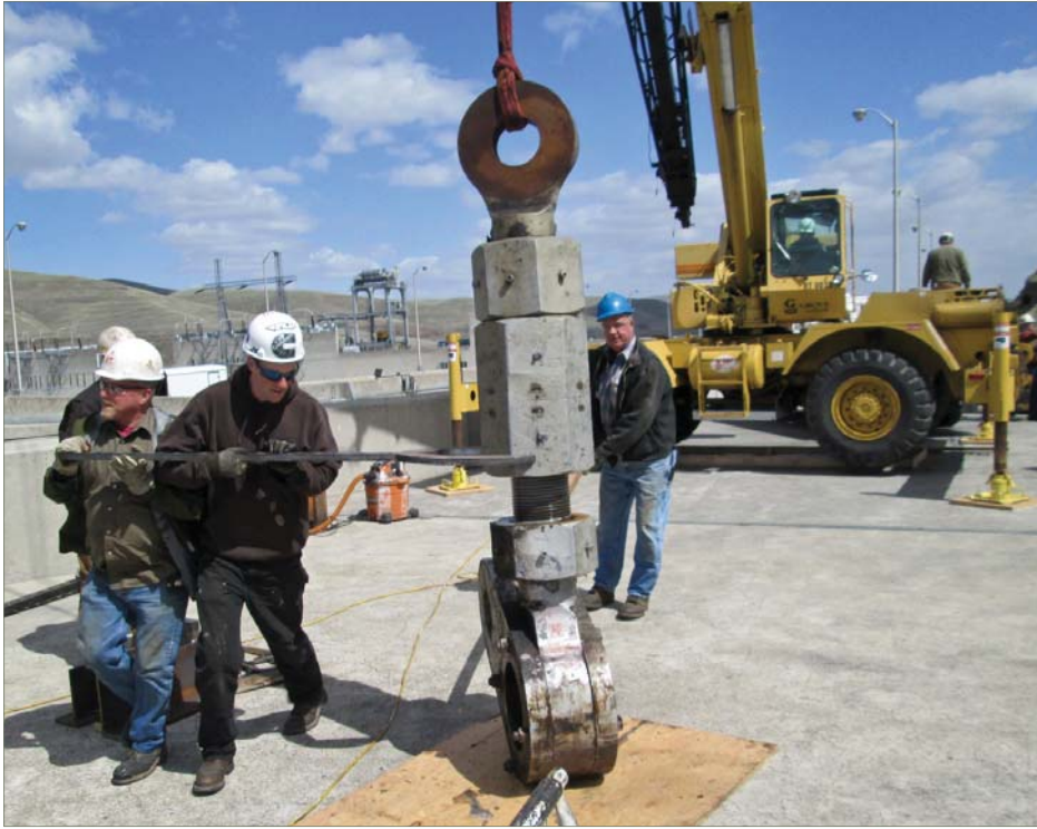
Above: Contractor workers take apart the old, cracked gudgeon arm assembly. The pieces were sent to a metallurgy laboratory for a failure analysis. Above, right: Little Goose 118-foot tall, 334-ton miter gate. Below: The dewatered Little Goose navigation lock.
