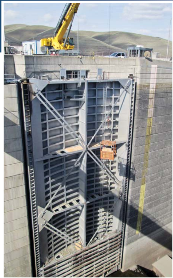
Above: Contractor workers take apart the old, cracked gudgeon arm assembly. The pieces were sent to a metallurgy laboratory for a failure analysis. Above, right: Little Goose 118-foot tall, 334-ton miter gate. Below: The dewatered Little Goose navigation lock.
