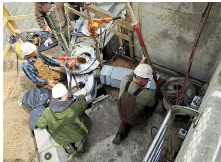
Above: Workers use an air-arc cutter to remove the 50-year-old pins. Above, center: Contractor workers used liquid nitrogen to shrink the new, bronze bushing, allowing it to fit into the new navigation lock gate gudgeon arm assembly. Right: Contractor workers at Little Goose Dam remove components of the cracked gudgeon arm assembly on top of the navigation lock's south gate leaf.
