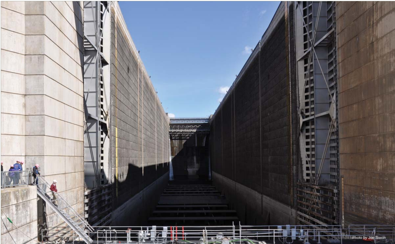
Above: Contractor workers take apart the old, cracked gudgeon arm assembly. The pieces were sent to a metallurgy laboratory for a failure analysis. Above, right: Little Goose 118-foot tall, 334-ton miter gate. Below: The dewatered Little Goose navigation lock.
