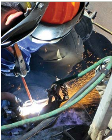
Above: Workers use an air-arc cutter to remove the 50-year-old pins. Above, center: Contractor workers used liquid nitrogen to shrink the new, bronze bushing, allowing it to fit into the new navigation lock gate gudgeon arm assembly. Right: Contractor workers at Little Goose Dam remove components of the cracked gudgeon arm assembly on top of the navigation lock's south gate leaf.
