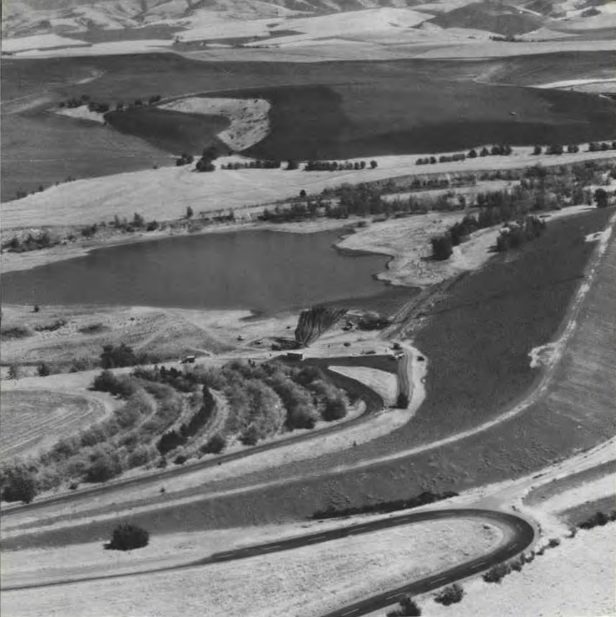
Mill Creek storage dam and lake
