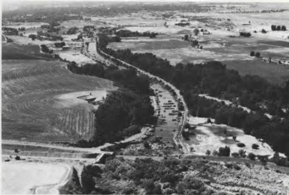
Stabilized Mill Creek channel
