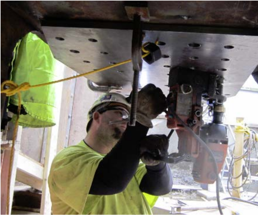
Pintle ball and receiver replacement
