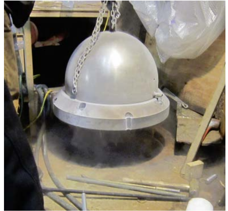
Pintle ball and receiver replacement
