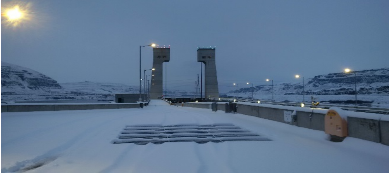
Adverse winter weather with ice build up in the lock chamber
