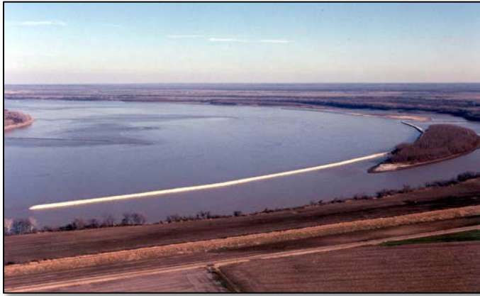
Figure 6. Dike on the Mississippi River
