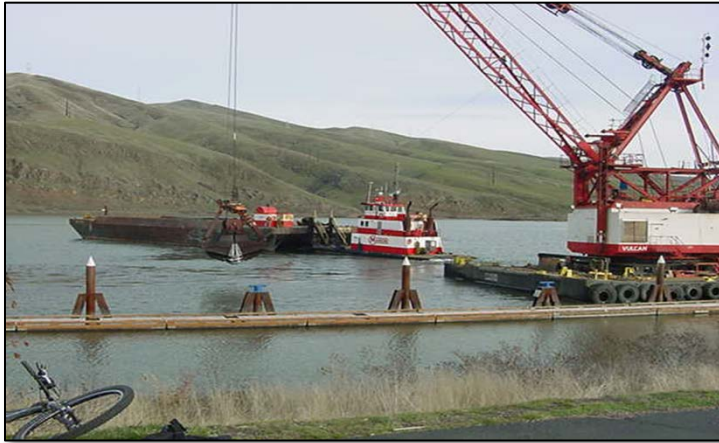
Figure 2. Dredging Operation on the Snake River.
