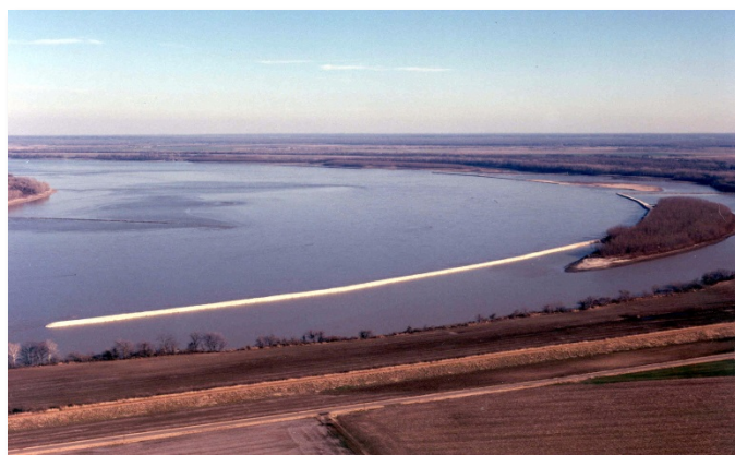
Figure 2-5. Dike on the Mississippi River
