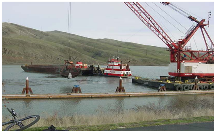
Figure 2-1. Dredging Operation on the Snake River
