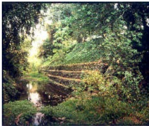
Figure 2-7. Gabion Baskets Installed for Slope Stabilization Along a Stream
