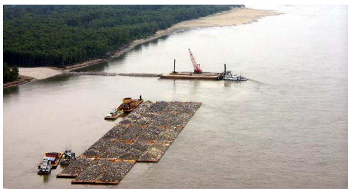
Figure 2-4. Dike Construction
