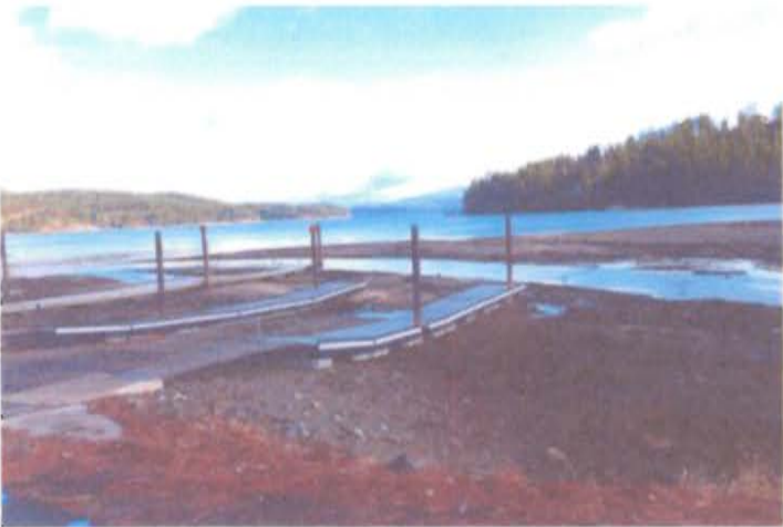
Photo 2: View out toward Mica Creek. Thalweg is visible at blue arrow; red arrow indicates accumulated sediments to be removed. Low water.
