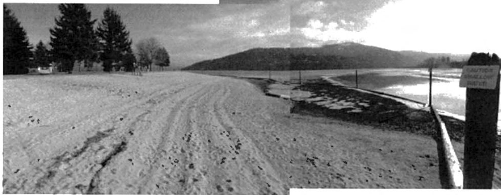
Photo 6. View east from south end City Beach. Shows erosion in bands, likely due to wave action and lake level fluctuation.
