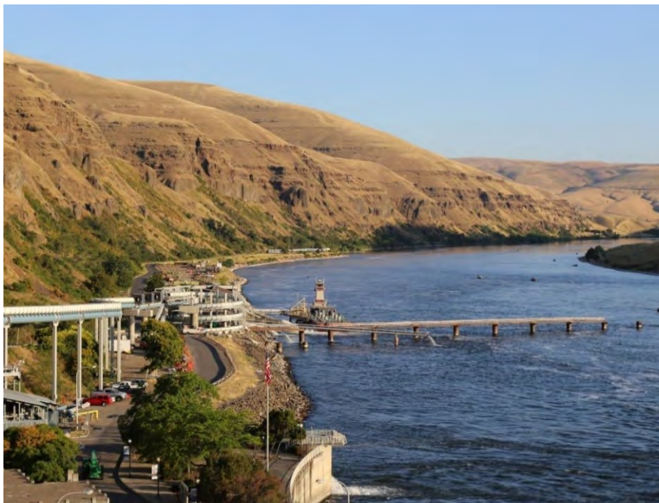
Figure 1-5. Lower Granite Dam New Juvenile Fish Facility, Bypass Pipe, and Fish Transportation Barge
