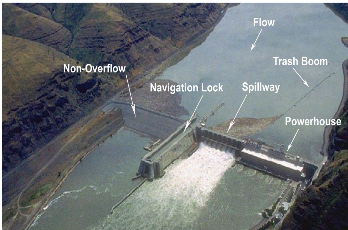
Figure 1-3. Lower Granite Lock and Dam Aerial View
