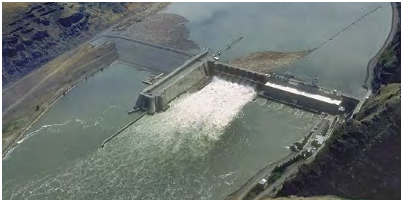
Figure 1-1. Lower Granite Lock and Dam
