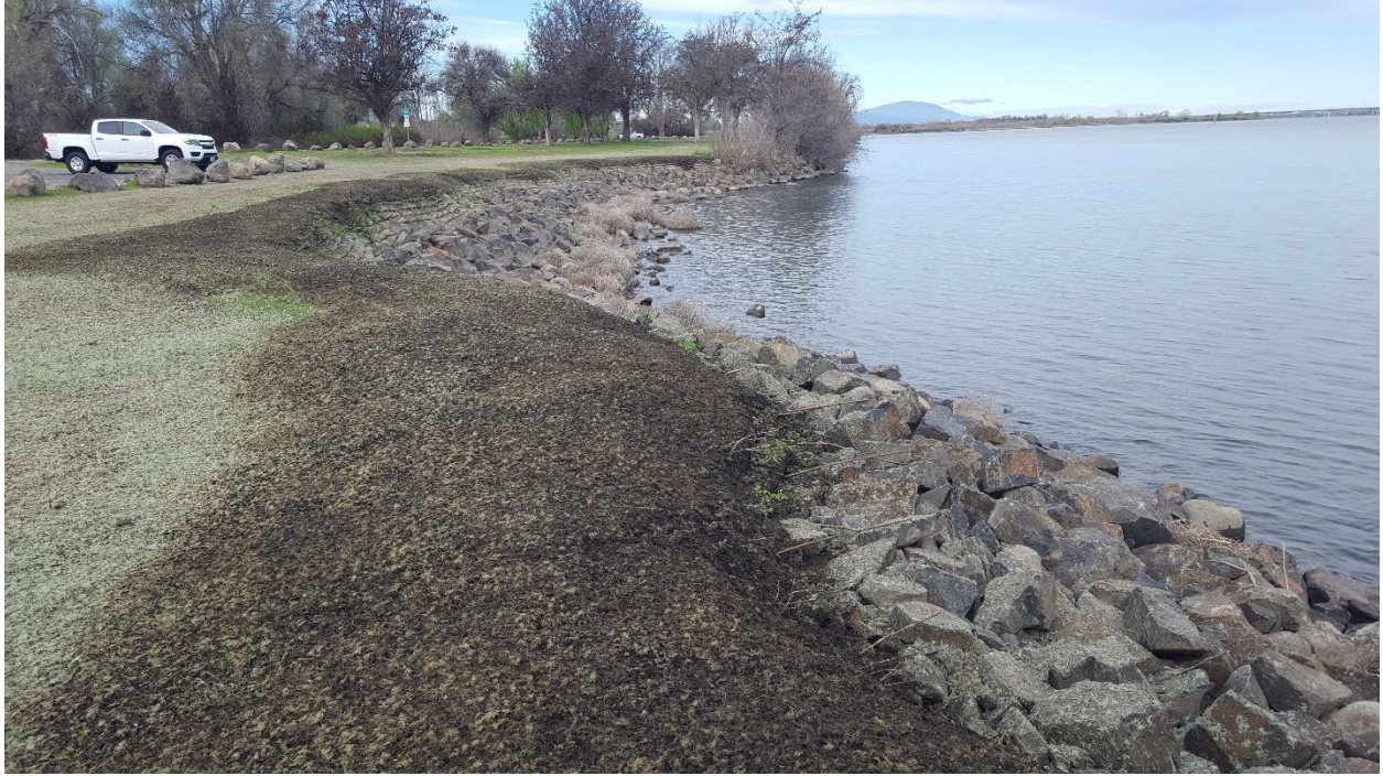
Figure 7. Example of a Rock Revetment along a River
