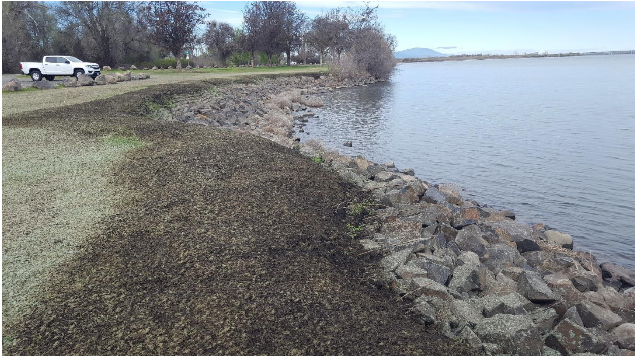
Figure 9. Example of a Rock Revetment along a River
