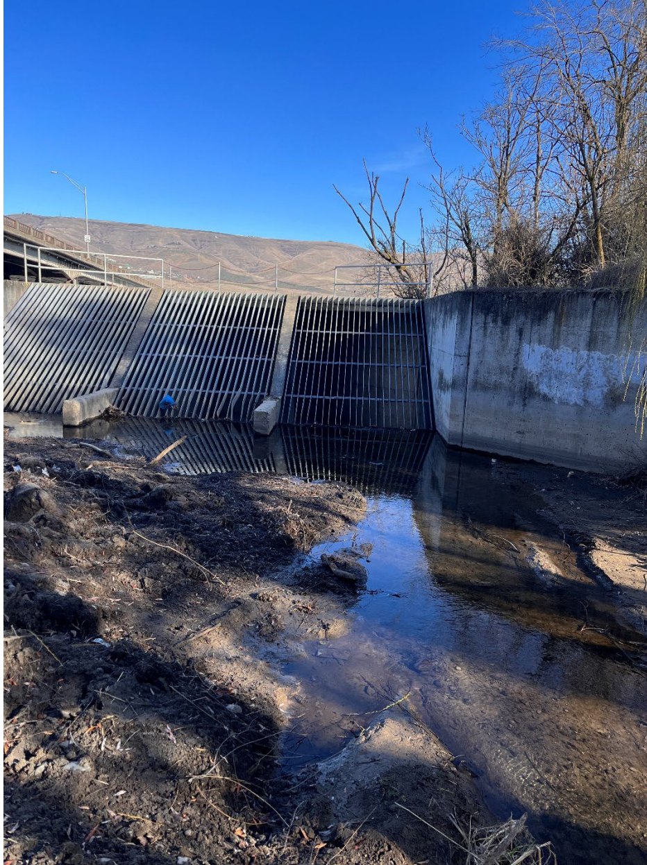
Figure 15. Intake Structure where the Stream Flows under Lewiston Levee System
