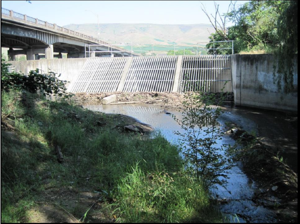
Figure 3. Area 380 Intake Structure with Accumulated Debris
