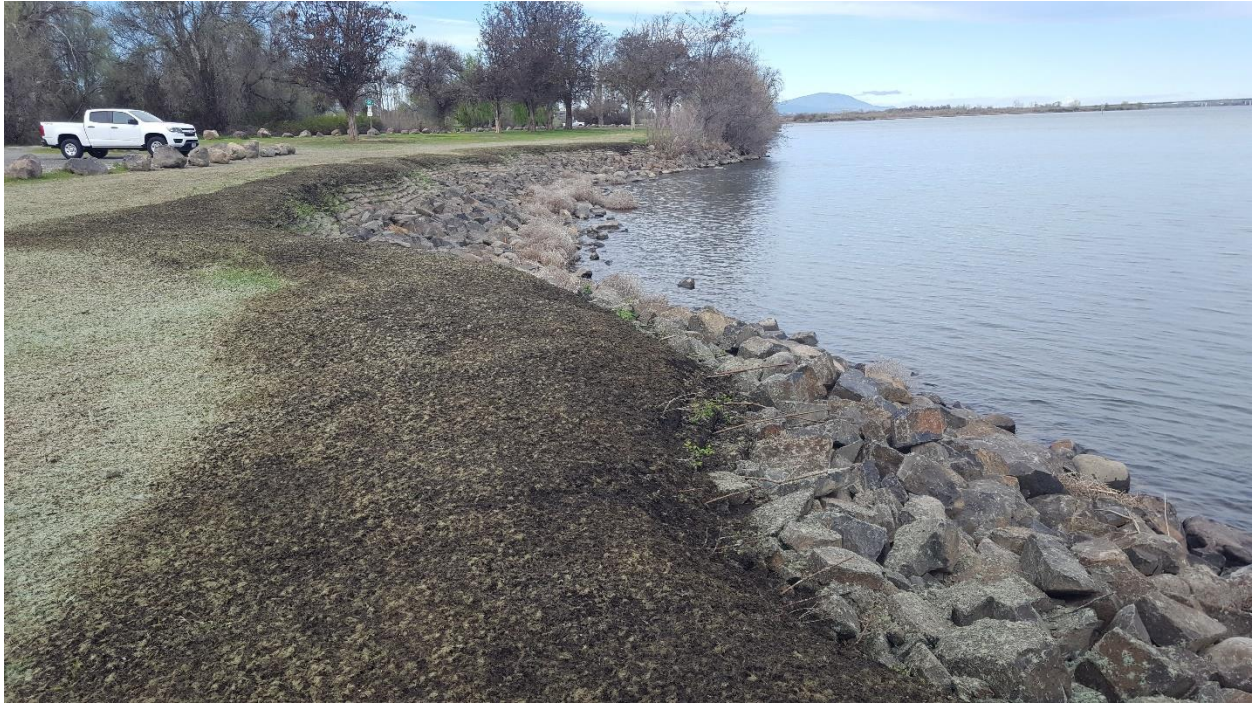
Figure 7. Example of a Shoreline Revetment along a River
