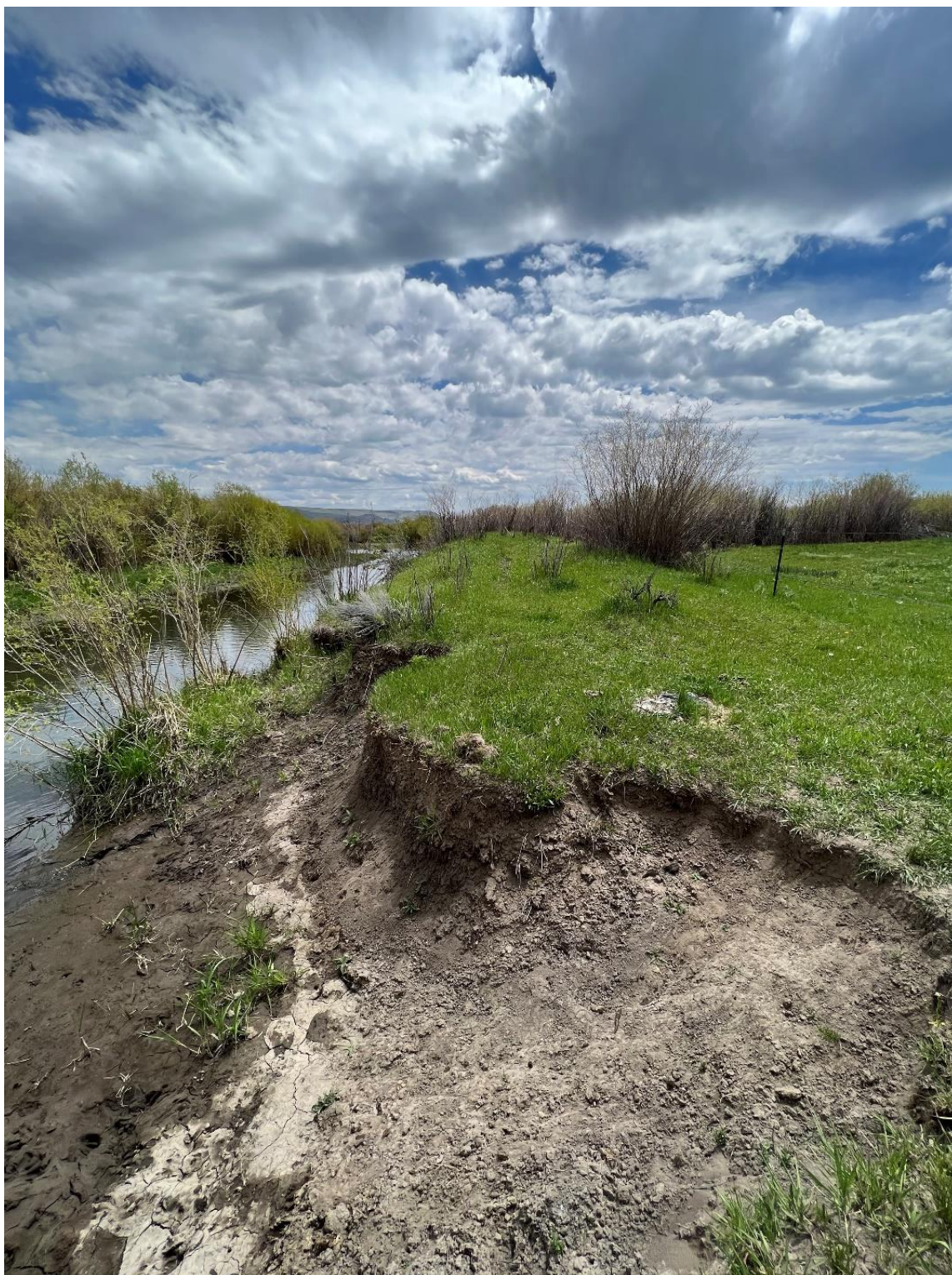
Figure 19. Berms that disconnect the Owyhee River from its adjacent floodplain.
