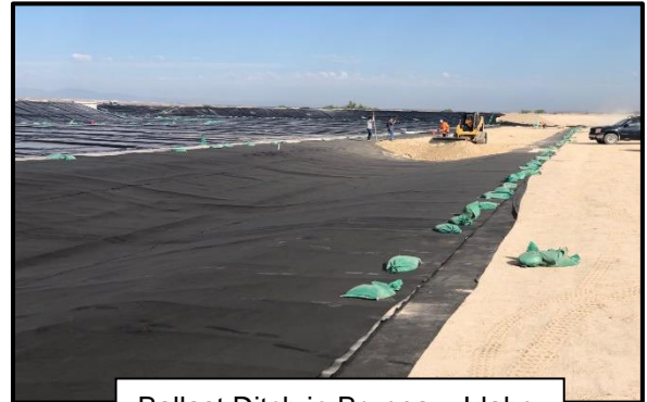
Ballast Ditch in Bruneau, Idaho
