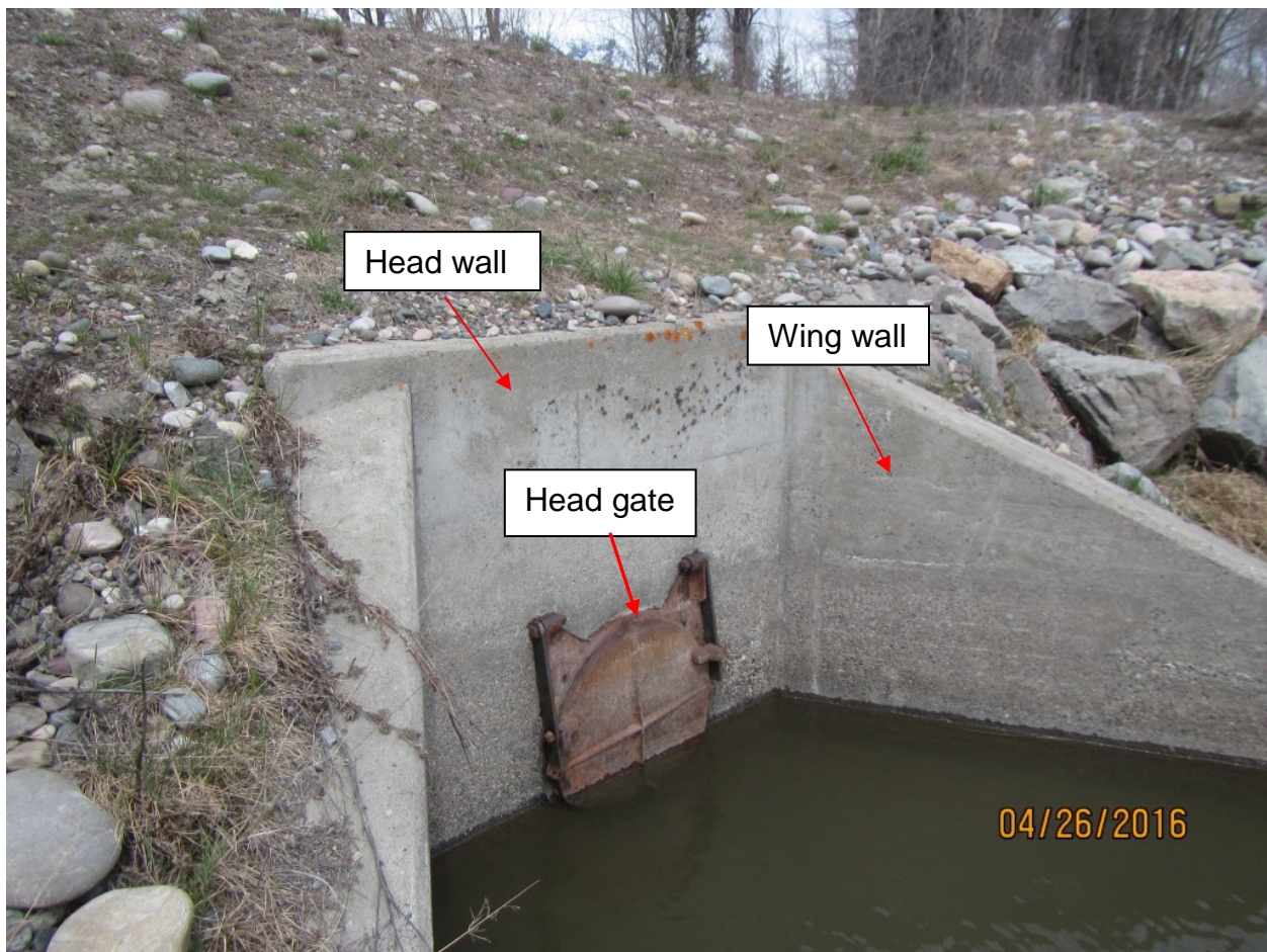
Figure 2-4. Flapper-type head gate on drainage culvert.
