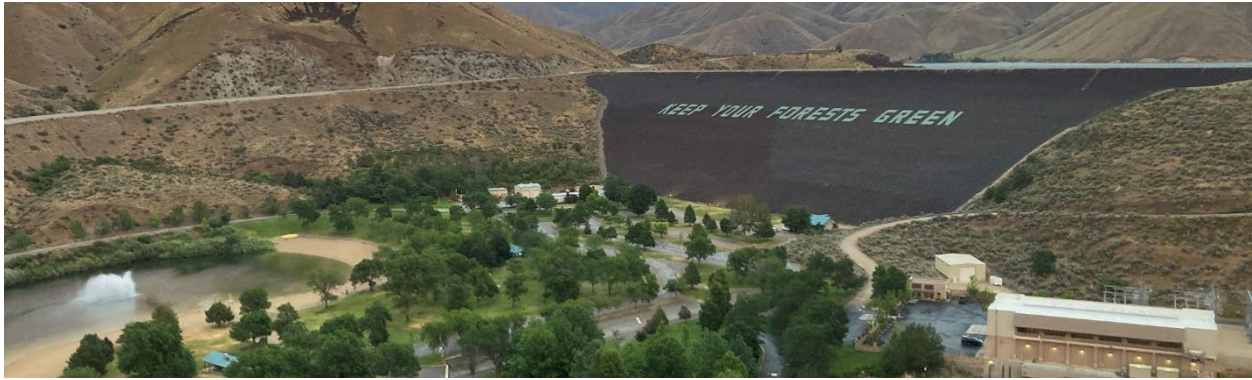
Figure 3-1: View of Luck Peak Dam, Exhibiting the Rolled Earth and Gravel Filled Dam
