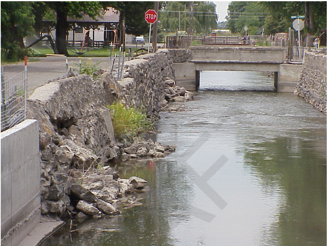
Figure 2 - Damaged section of wall between Main Street and Idaho Street.
