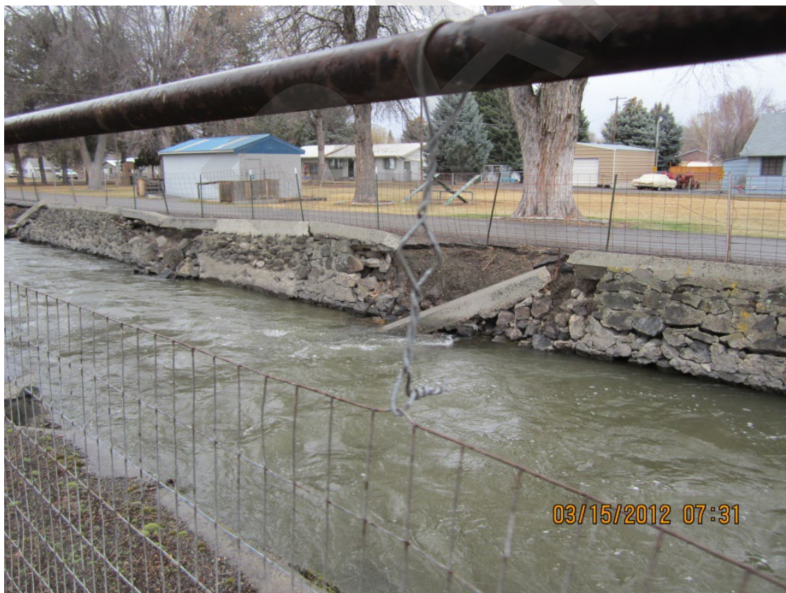
Figure 1. Example of Failing Walls on the Little Wood River at Gooding, Idaho
