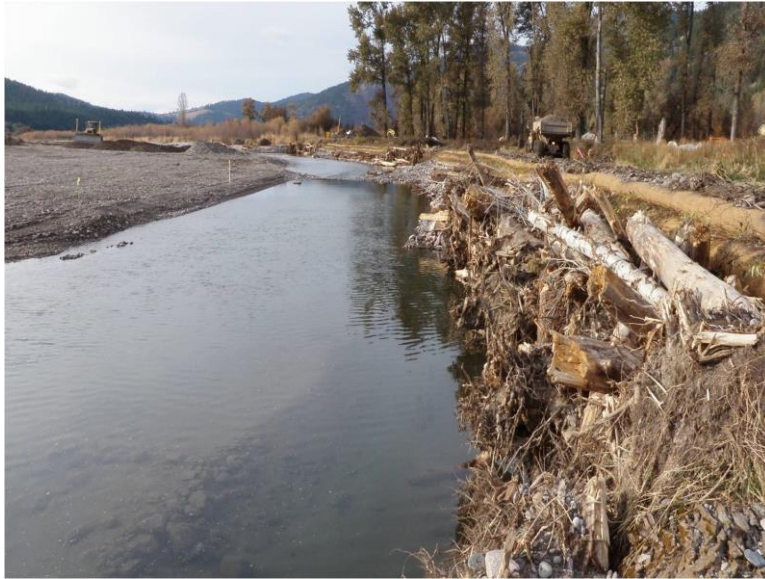
Figure 3-6. Example Meander Sequence with Integrated Instream Wood Structures
