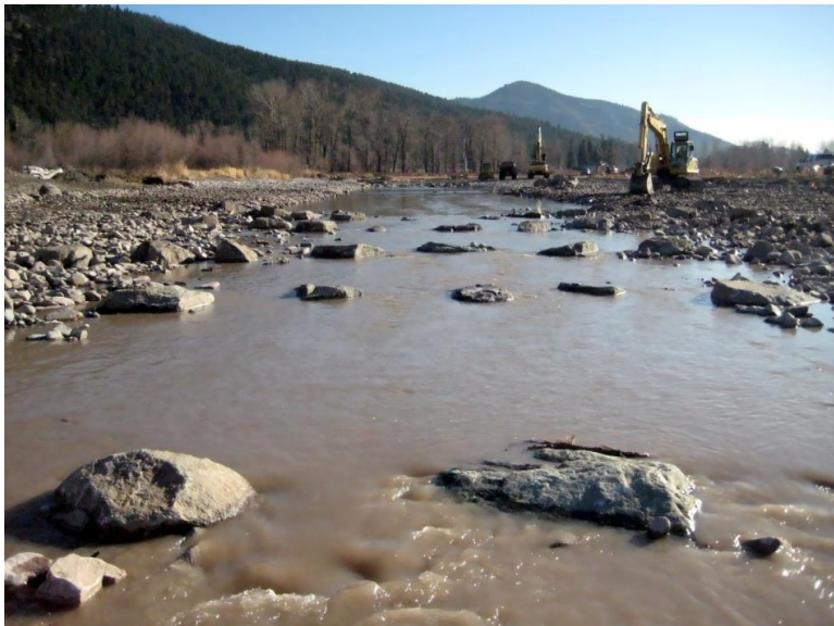
Figure 3-5. Example Instream Roughened Riffle with Boulder Grade Control
