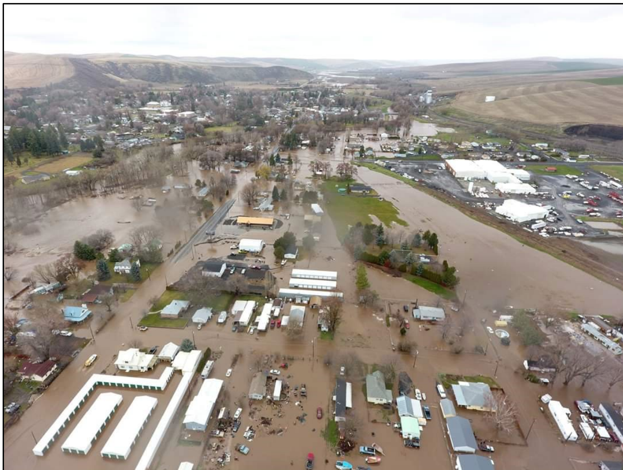
Figure 3. Overland flooding originating in nearby Columbia County as it inundates everything in its downstream path.
