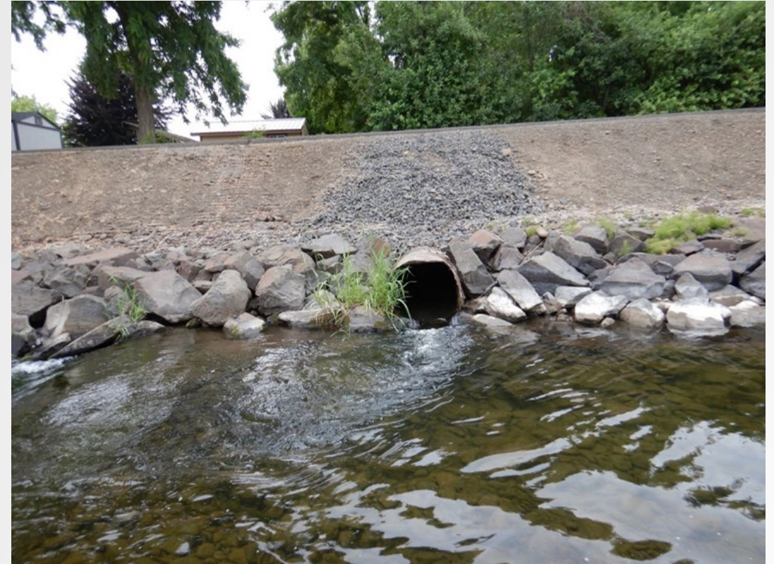
Titus Creek Culvert
