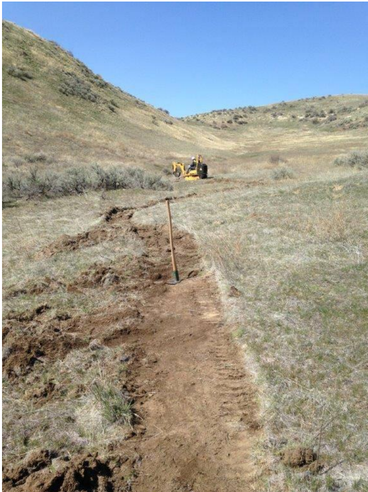
Figure 21 Easy trail finishing behind the Single Track 240 with a hand tool.
