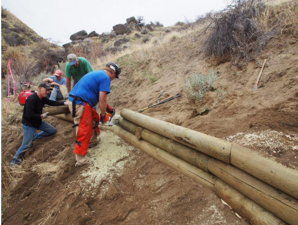
Figure 7 Example using pressure treated logs and rebar to build a retaining wall. There is a fourth layer of logs not seen that is below the surface and anchoring the wall with 3' of rebar below.
