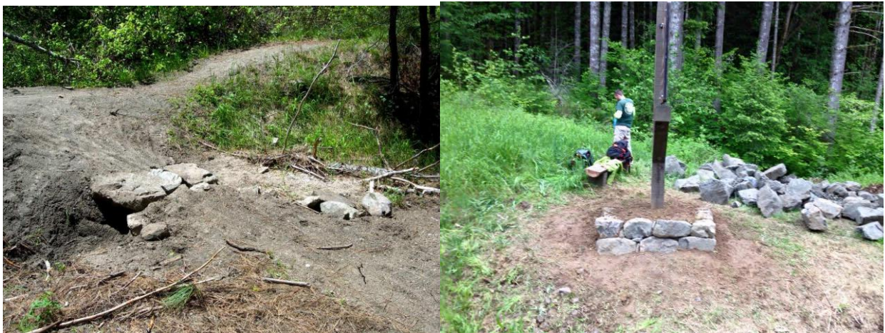
Figure 17 A rock culvert built by SWIMBA on the East Side Trail System and a rock retaining wall around a sign done as part of a Professional Trail builders class on “Building with Rock” taken by SWIMBA trail leaders.
