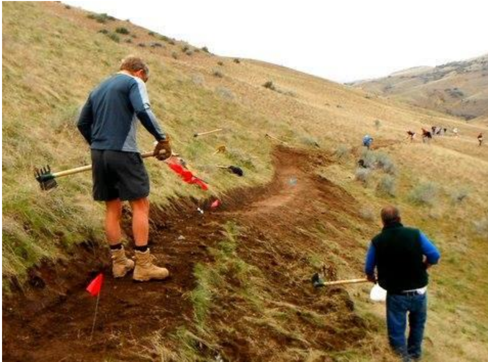
Figure 3 Example of incorporating grade reversals to get water to shed off the trail and avoid erosion
