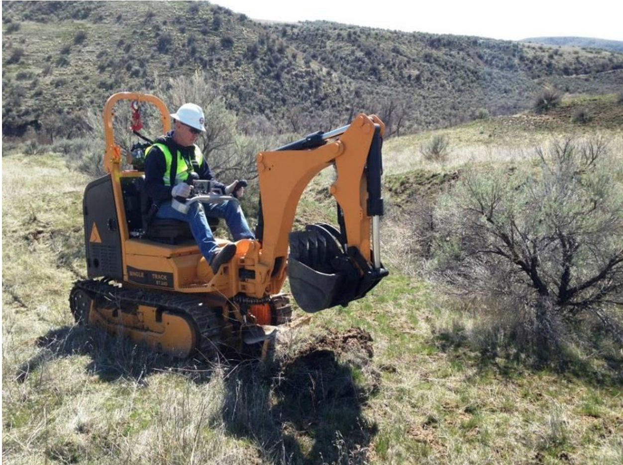
Figure 19 First ground breaking with the new Single Track 240 on Chutes and Ladders at Avimor
