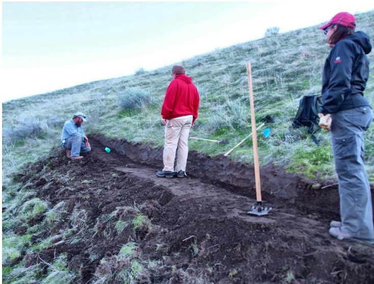
Figure 1 Using a McLeod to check out slope of the trail.
