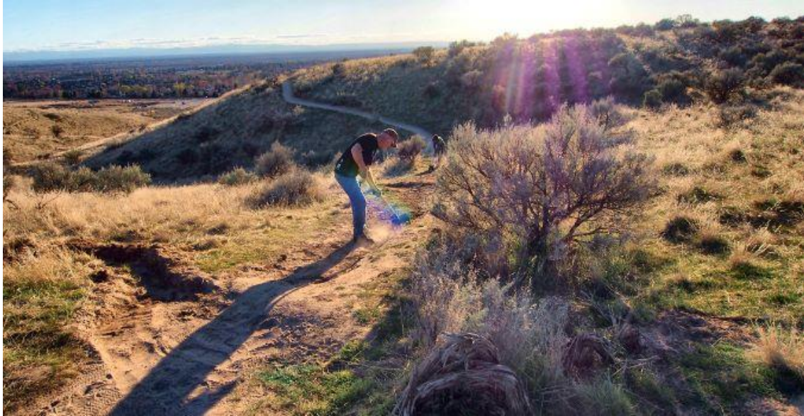
Figure 5 Where grade reversals weren't incorporated into a trail sometimes it's necessary to put in water bars to help direct the water off the trail as can be seen by the SWIMBA volunteer at the Eagle Bike Park.
