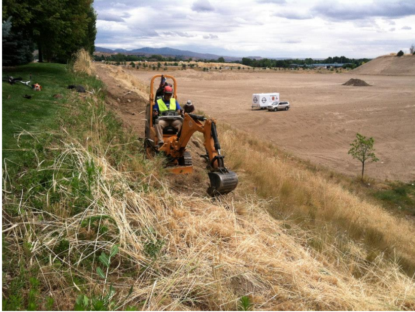
Figure 20 Cutting in a new trail at Guerber Park for the City of Eagle.
