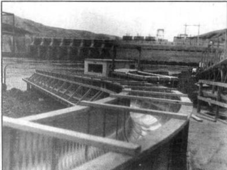
*Construction of juvenile fish bypass system model at Lower Granite,
