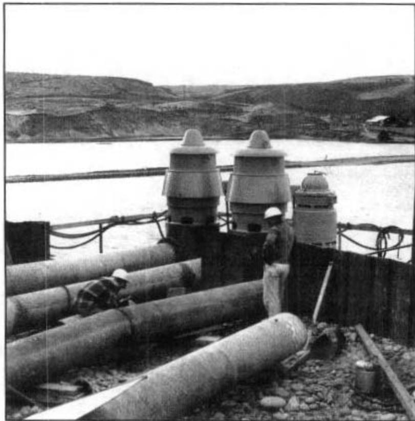
*Installation of south shore cofferdam pumps used to keep work area dry during dam construction, December 1956.*
