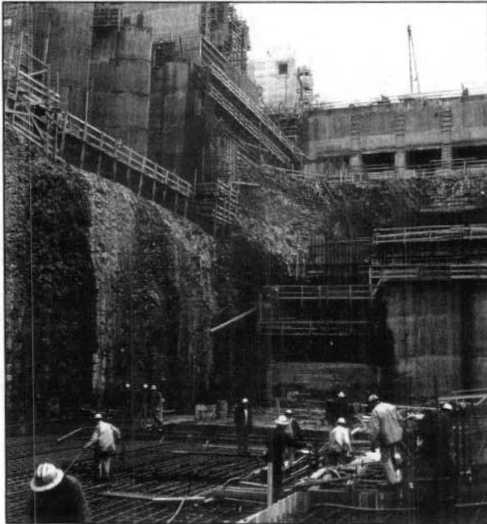
*Draft tube area, powerhouse and non-overflow section under construction, January 1958.*
