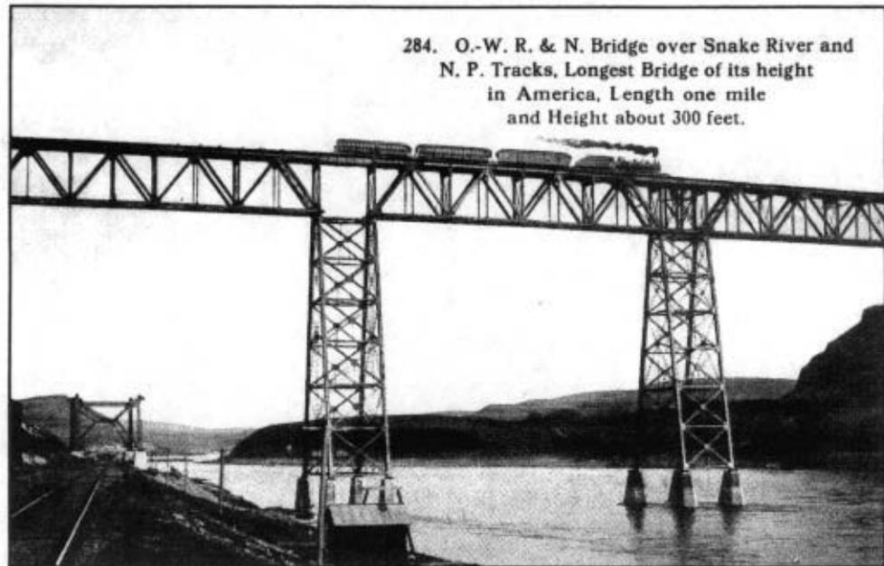
284. O.-W. R. & N. Bridge over Snake River and N. P. Tracks, Longest Bridge of its height in America, Length one mile and Height about 300 feet.
