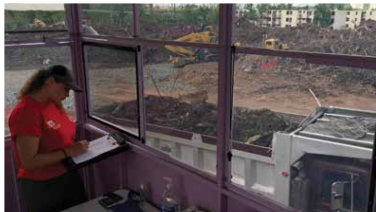
Left: A Debris Quality Assurance Inspector, Jackie Roy, rates a load of storm debris delivered by a contractor truck to the Toa Baja Landfill. Debris QAs ensure contractor invoices accurately reflect work performed. QA's often perform dual roles, rating loads as well as inspecting and certifying trucks hauling debris for USACE contractor Keith Hyde. Above: A Debris Quality Assurance Inspector rates a load of vegetation received at the Los Alamos temporary debris reduction site where grinders reduce woody debris into mulch which will serve beneficial use elsewhere on the island.
