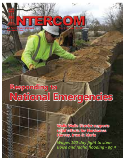
Corps builds levee to prevent Boise River flooding near Eagle Island, Idaho. US Army Corps of Engineers photo)
