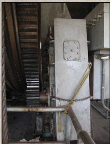
Gear boxes to be replaced at Lower Monumental Lock and Dam.
