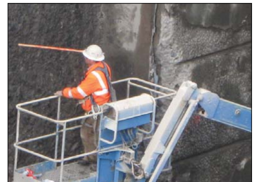
Progression of construction on Lower Monumental's lock wall. Workers removed 700 tons of concrete from the lock wall.
