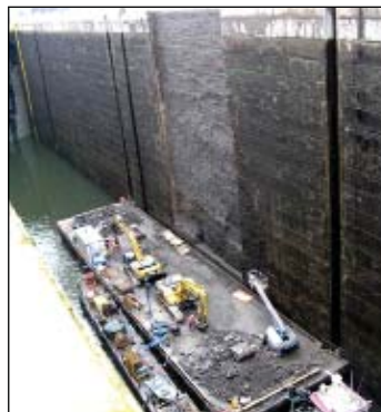
Progression of construction on Lower Monumental's lock wall. Workers removed 700 tons of concrete from the lock wall.
