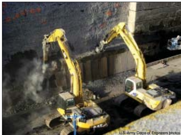
U.S. Army Corps of Engineers photos
