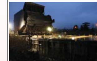
The Removable Spillway Weir was the first type of spillway weir—a fixed, semi-permanent structure that occupies one spillway bay. Air is added or removed from tanks incorporated into the structure to either raise it up to its operational position in the spillway, or lower it to its stowed position on the riverbed.
