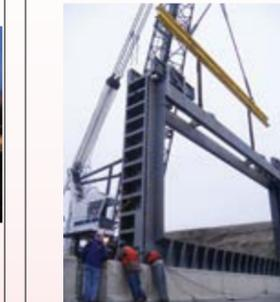
2nd Generation Spillway Weirs were installed at Little Goose and McNary Dams. They use a gantry crane to change weir segments to adjust the weir's height to change the amount of water flowing over it.
