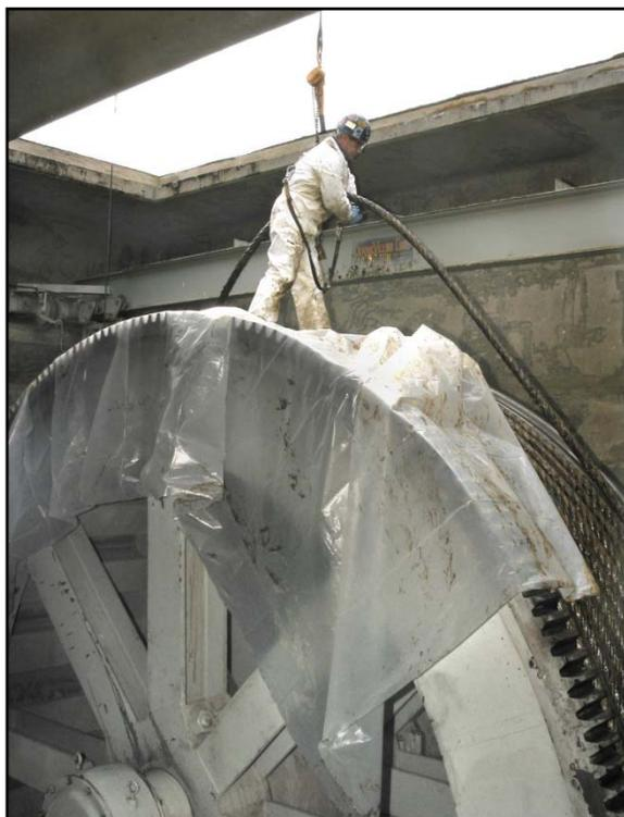
**Ice Harbor Lock and Dam** – New operating machinery for the downstream gate at Ice Harbor is a very high priority for the Walla Walla District. Critical components of the machinery and control systems require replacement during the extended closure.
