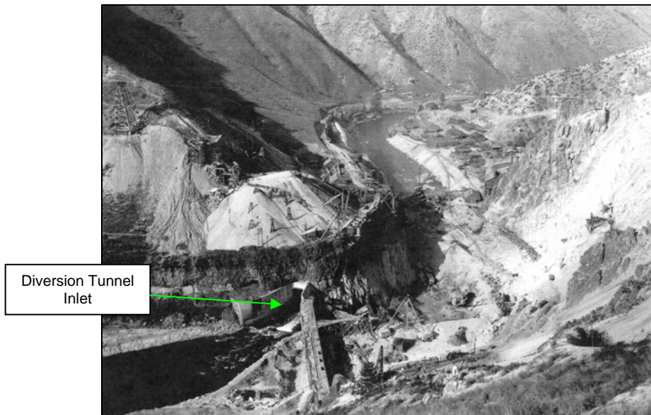
Figure 2. Diversion Tunnel During Construction of Arrowrock Dam
