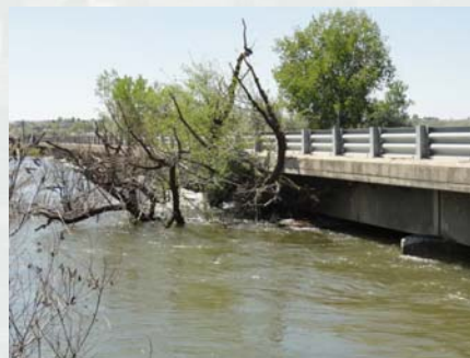
Highway 95 Bridge near Parma, ID at approx. 8,000 cfs
