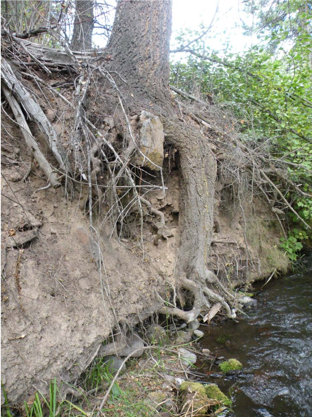
Figure 4. Streambank erosion on Charley Creek near Asotin, WA.
