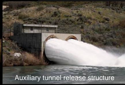
Auxiliary tunnel release structure
