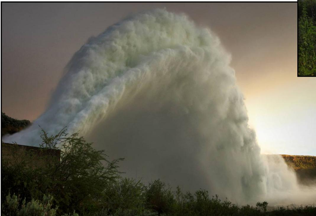
The Rooster Tail only uses water from large releases required for flood risk management that exceed powerhouse capacity, thus no water is wasted for the display. It occurred daily until 1986 when construction of the Lucky Peak Power Plant Project started.
